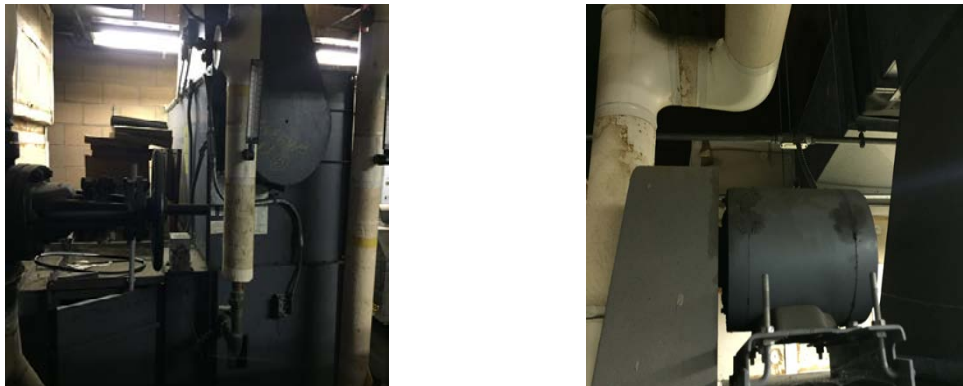
Image 16: AHU (HV-1) - Maintenance Garage Building
