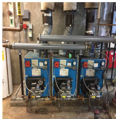
Image 18: Oil-Fired Hydronic Boilers – Administration Building
