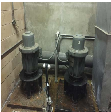
Image 24: 15 hp Pump motors and Flow Monitoring Control Panel
