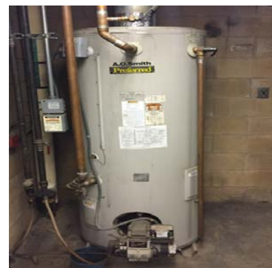
Image 26: Vanguard Electric Water Heaters and an A. O Smith Oil-Fired Water Heater
