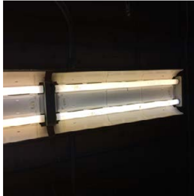
Image 13: Typical Interior Fluorescent T12 Fixtures
