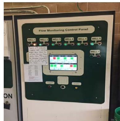
Image 24: 15 hp Pump motors and Flow Monitoring Control Panel
