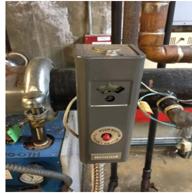
Image 19: Hot Water Pump and Aquastat – Administration Building
