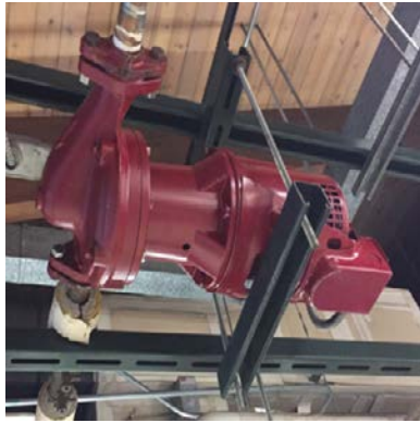
Image 19: Hot Water Pump and Aquastat – Administration Building
