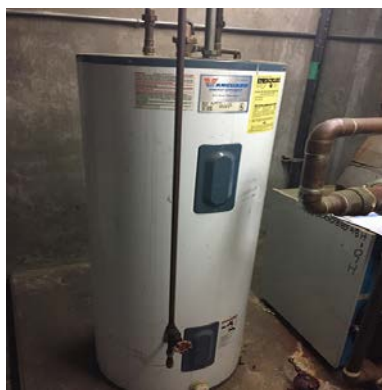
Image 26: Vanguard Electric Water Heaters and an A. O Smith Oil-Fired Water Heater
