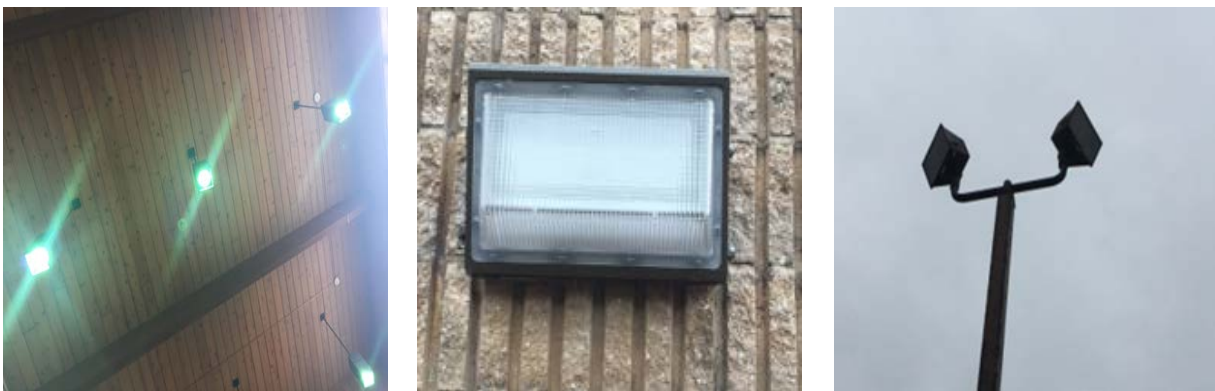
Image 11: Mercury Vapor and Exterior Fixtures
