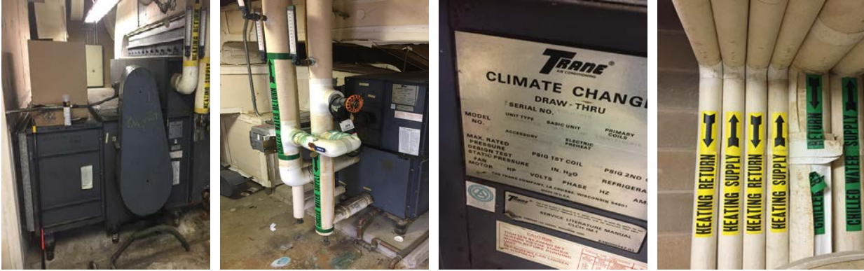
Image 14: A Multi-Zone and A Single Zone AHU – Administration Building
