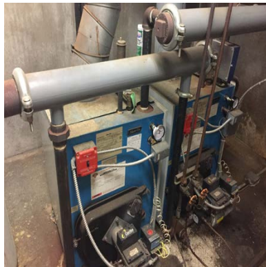
Image 20: Hot Water Heating System - Nursery Building
