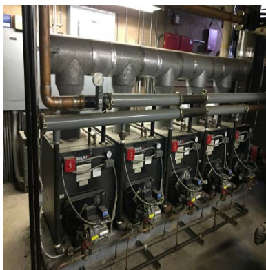
Image 21: Hot Water Heating System - Maintenance Garage Building
