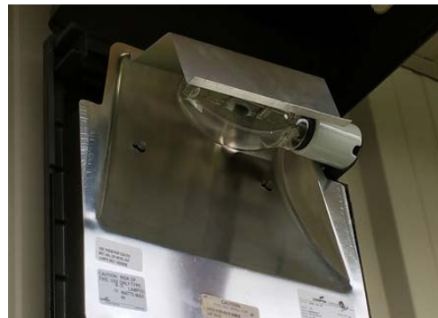
175 Watt Metal Halide
