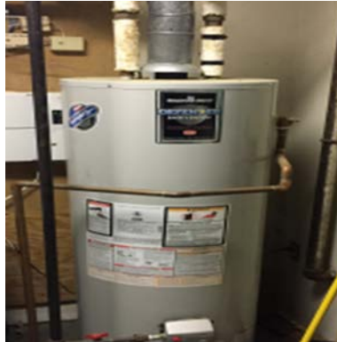
Image 7: Domestic hot water system
