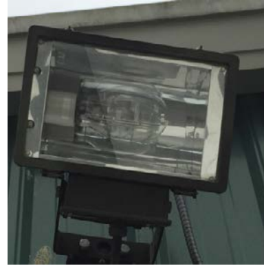
Image 4: Wall Mounted Metal Halide Fixtures - Main Building
