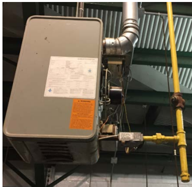
Image 8: Gas-Fired Unit Heater and Local Thermostat
