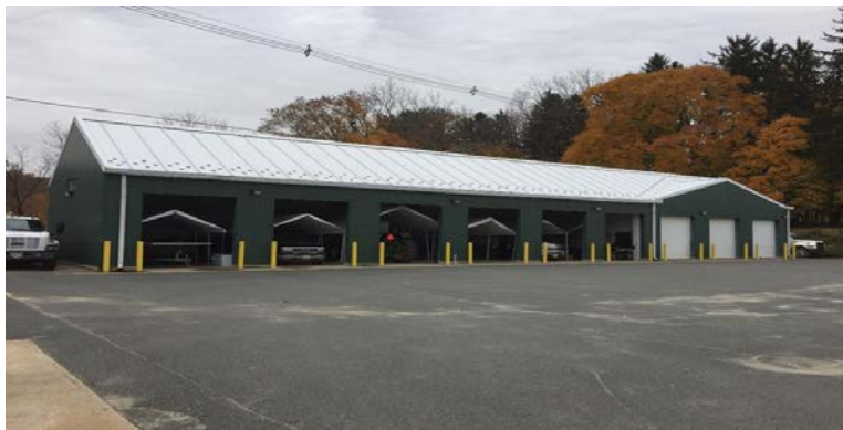
Image 2: Maintenance Garage Building Envelope
