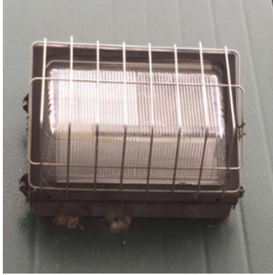
Image 4: Wall Mounted Metal Halide Fixtures - Main Building
