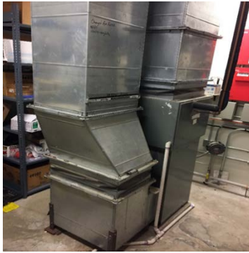
Image 7: Gas-Fired Furnace and Rheem Condensing unit
