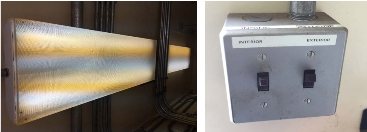
Image 2: Interior Linear T12 Fixtures
