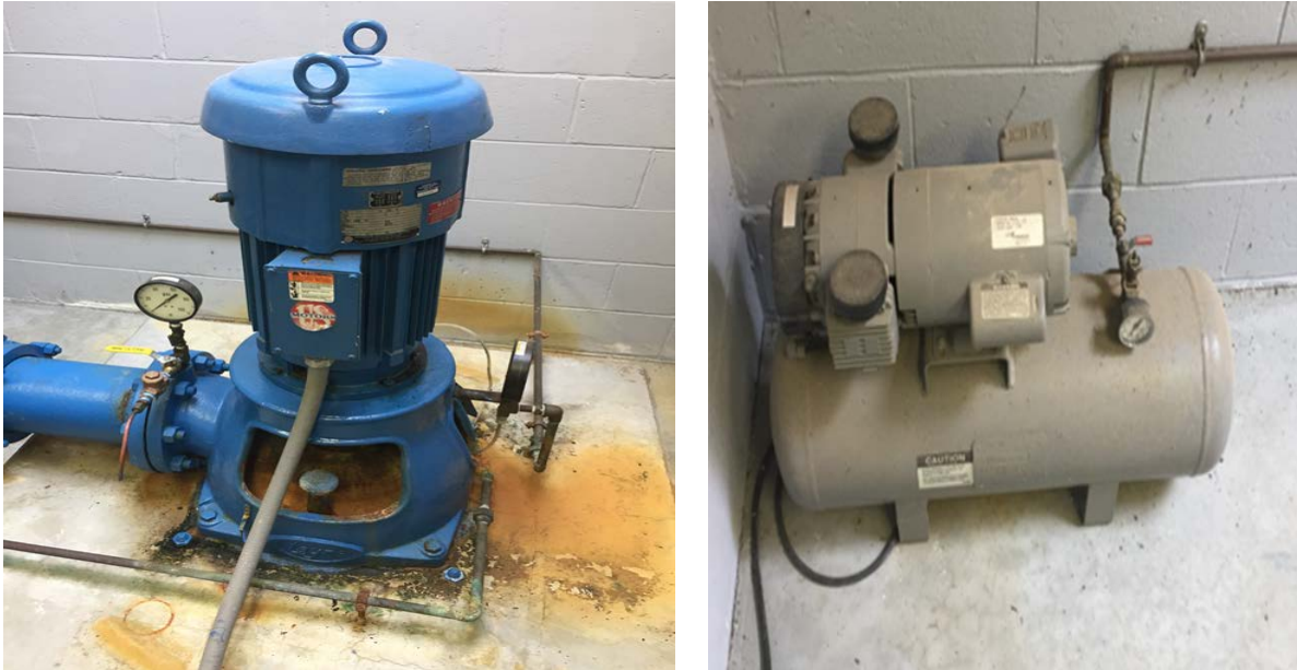
Image 3: Well Pump & Compressed Air Pump
