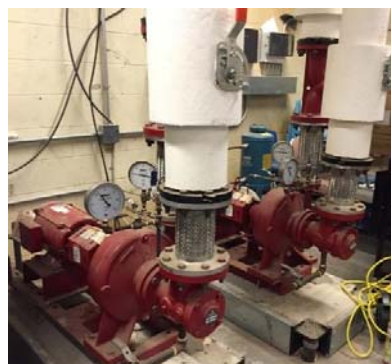
Hot Water Pumps on VFDs
