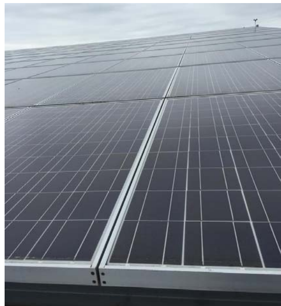
Rooftop Solar Array
