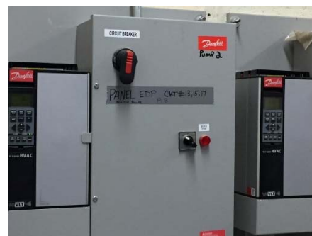
Hot Water Pumps on VFDs
