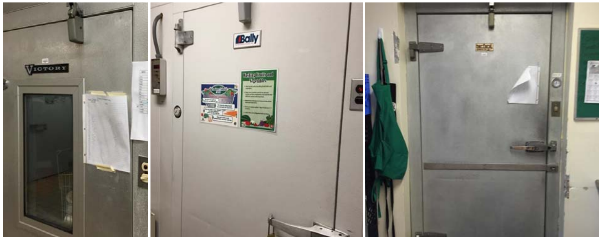
Walk-In Coolers and Freezers
