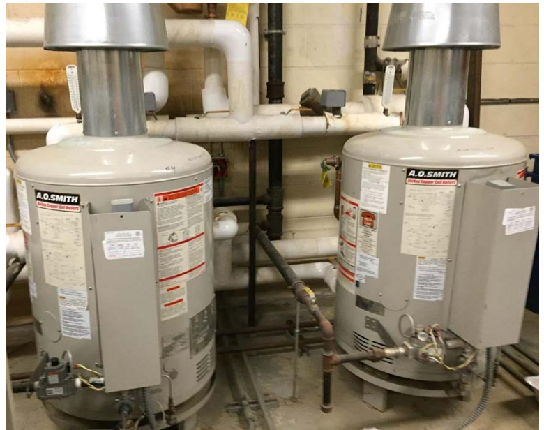
Domestic Hot Water Heaters
