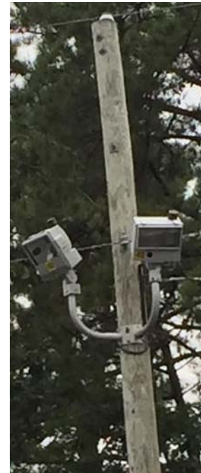
Parking Lot Lighting
