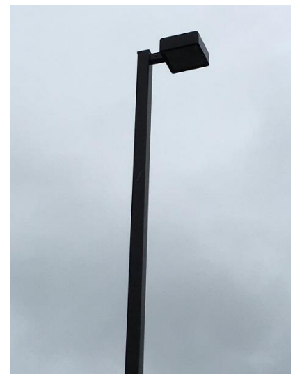
Box-Type Mercury Vapor Pole Lighting in Parking Lot
