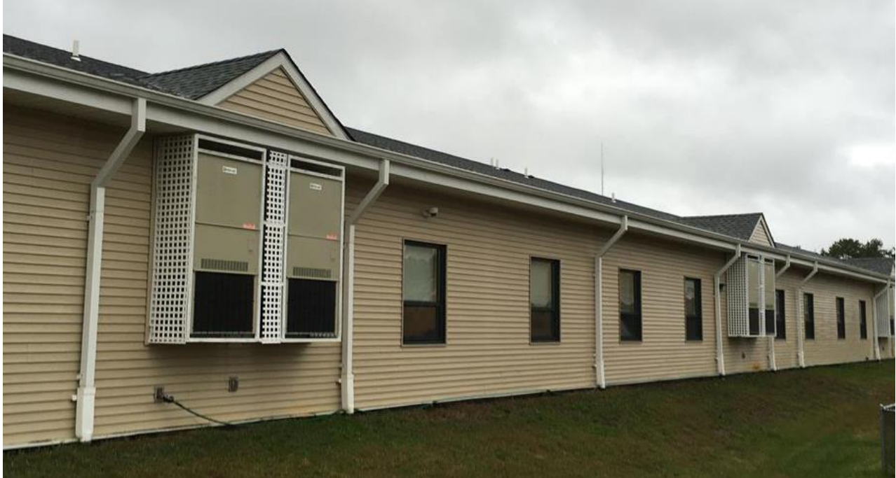
Rear Facade of Building Showing Vinyl Siding, Windows, and Roof
