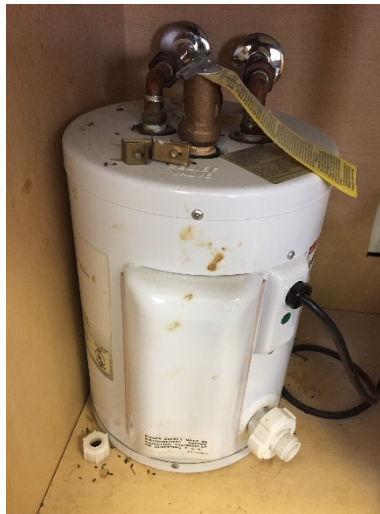
Image 7: Domestic Water Heater
