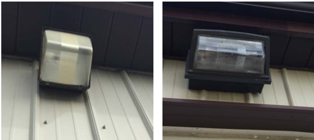
Image 3: Metal Halide Fixtures
