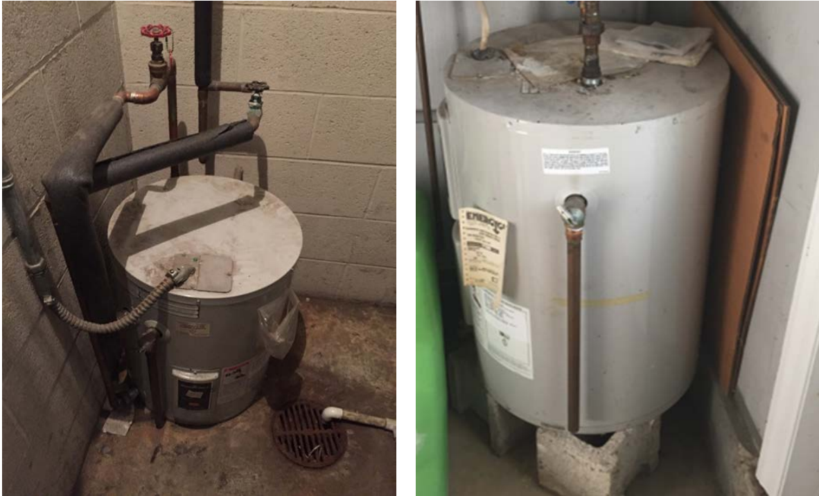
Image 10: 19-Gallon & 30-Gallon Electric Water Heaters
