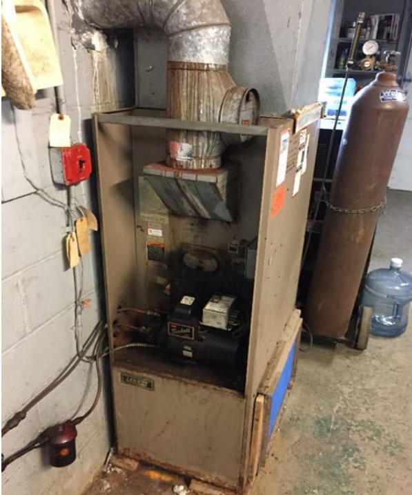
Oil-Fired Furnace and Exterior Oil Tank - Old Maintenance Building
