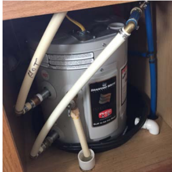
Image 5: Electric Water Heater & Restroom Sink
