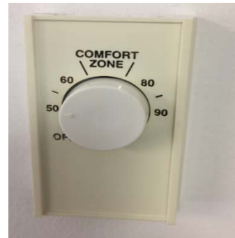
Image 4: Electric Baseboard Heaters & Thermostat
