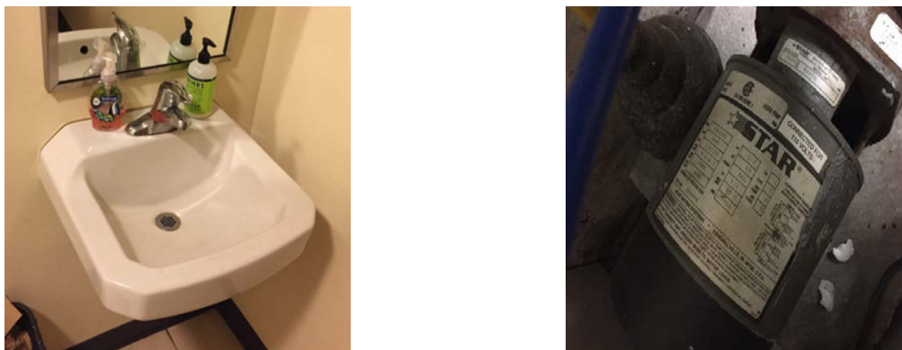
Image 6: A Restroom Sink & Well Pump
