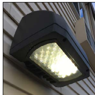
LED Wall Packs
