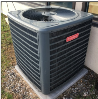
Goodman AC condensing unit
