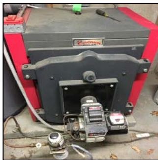
Hot water boiler
