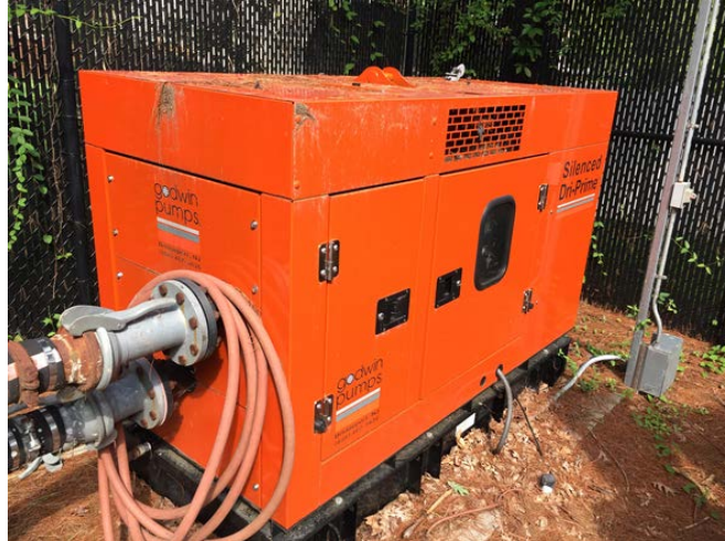
Image 3: Diesel-Fired Bypass Pump
