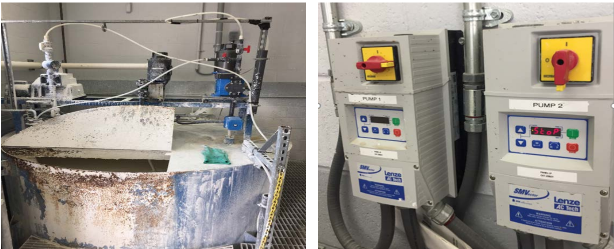
Image 8: Lime & Mixing Pumps
