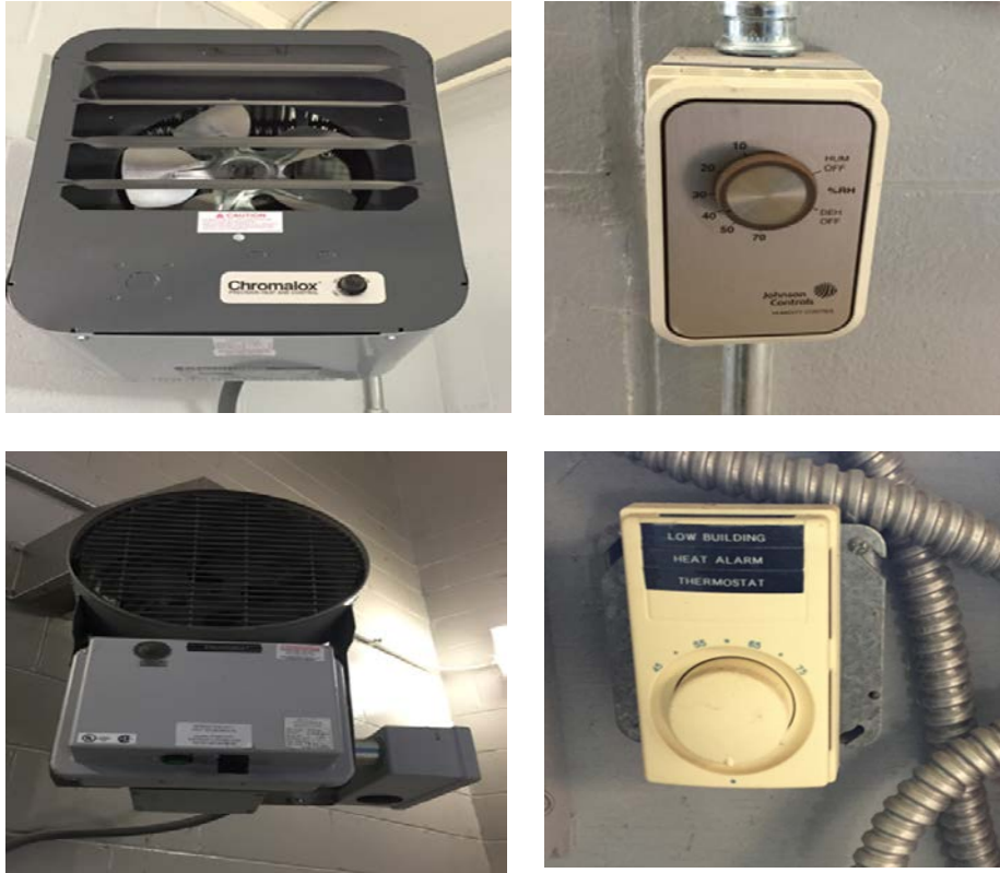
Image 6: Space Heating System
