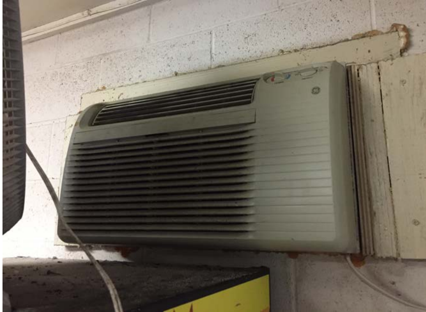
Image 4: PTAC In Kitchen
