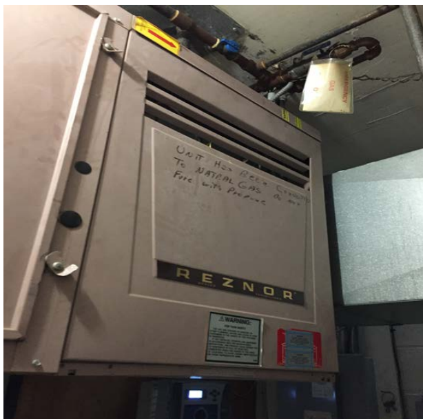
Image 5: Gas-Fired Furnace
