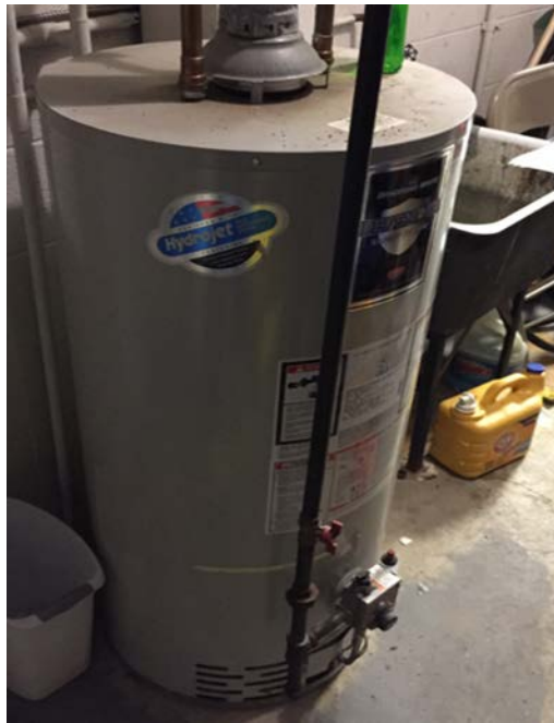
Image 6: 40 Gallon, Gas-Fired Water Heater
