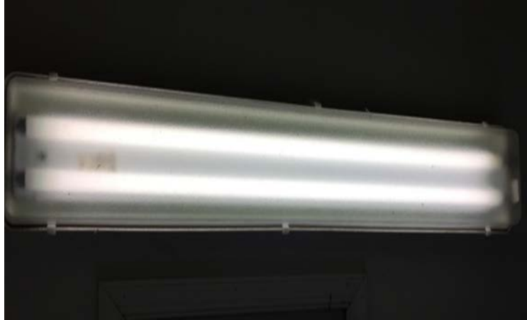
Image 2: Interior Fluorescent T8 Lamps
