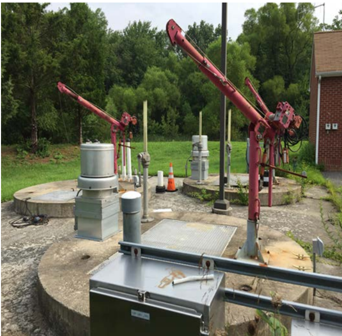
Image 5: Underground Pumps & Exhaust Fans
