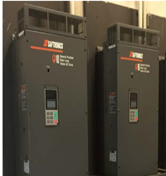
Image 4: Grinder Pump & Variable Frequency Drive Control Units
