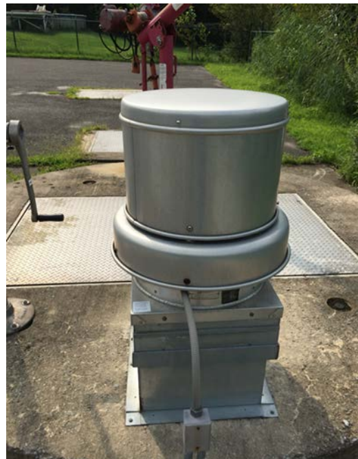
Image 5: Underground Pumps & Exhaust Fans
