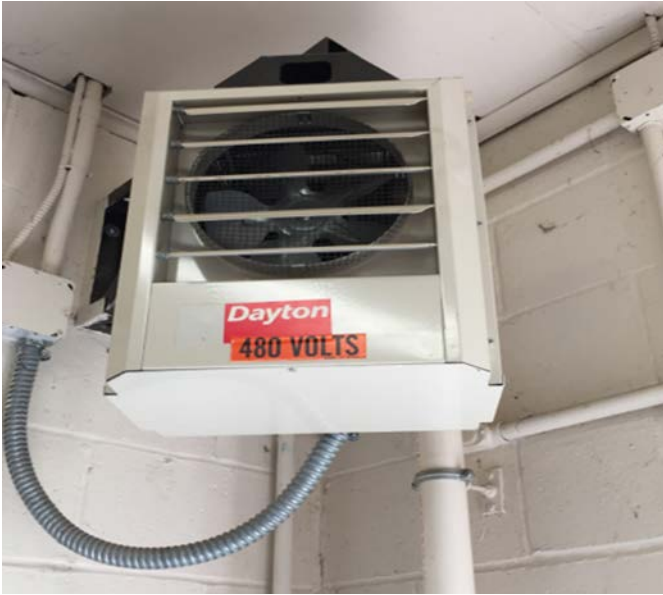
Image 6: Electric Resistance Heater
