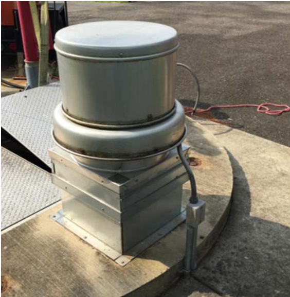
Image 5: Exhaust Fan & Thermostat Control
