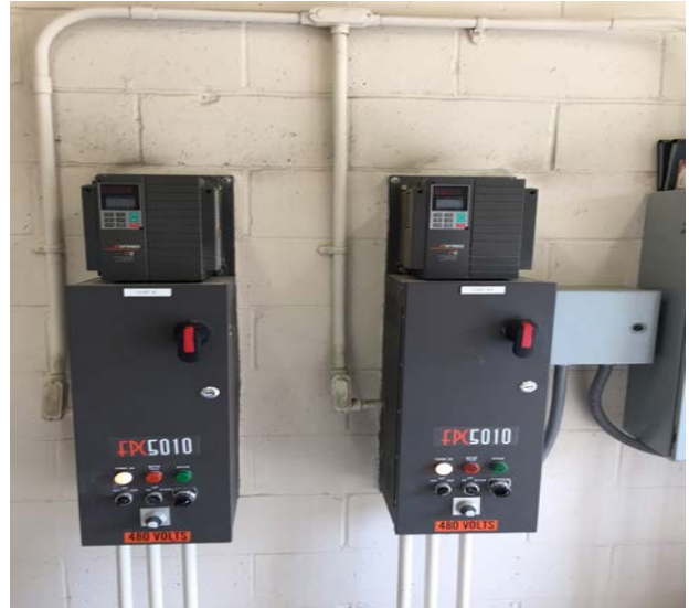
Image 4: Hydraulic Grinder & VFD Controls System
