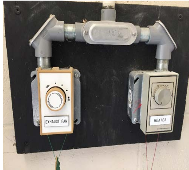
Image 5: Exhaust Fan & Thermostat Control
