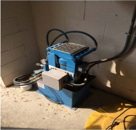
Image 4: Hydraulic Grinder & VFD Controls System
