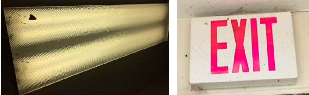
Image 2: Interior Lighting System
