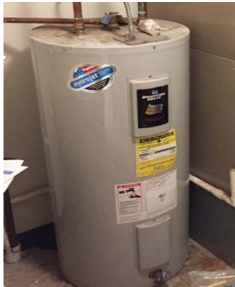
Image 6: 40 Gallon Electric Storage Tank Water Heater
