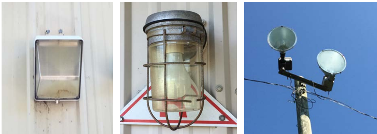
Image 3: Exterior Perimeter & Pole Mounted Fixtures
