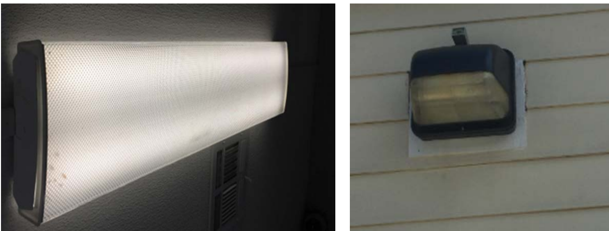
Image 2: Interior & Exterior Lights
