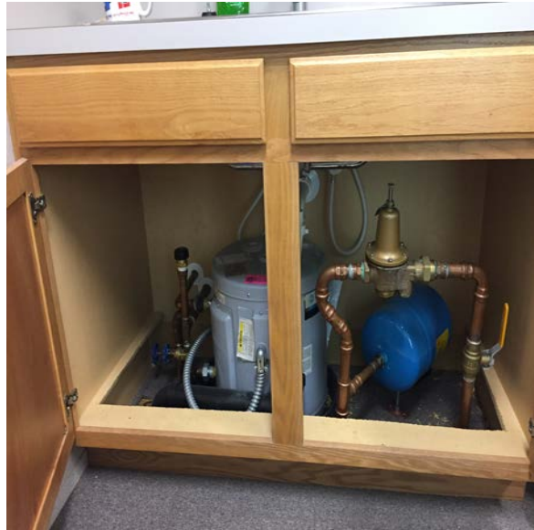
Image 4: Domestic Water Heater
