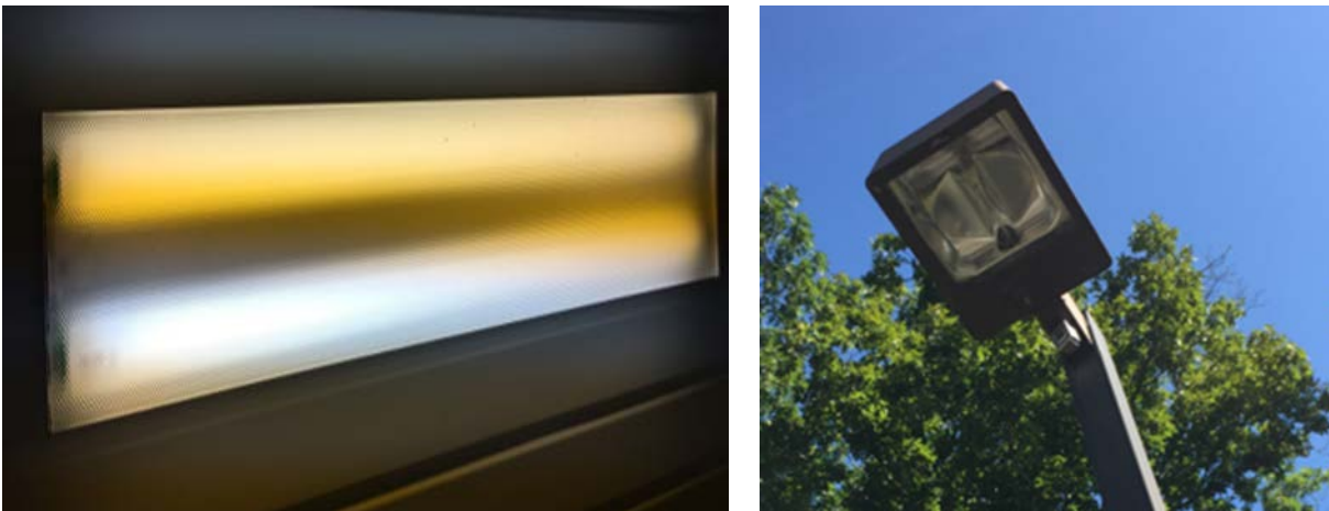
Image 2: Interior & Exterior Lights
