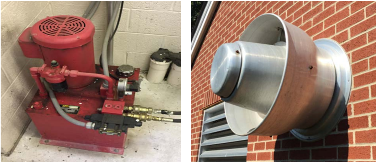
Image 3: Hydraulic Grinder Pump & Exhaust Fan
