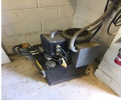
Image 5: Hydraulic Grinder Pump & Ground Mounted Exhaust Fan
