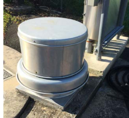
Image 5: Hydraulic Grinder Pump & Ground Mounted Exhaust Fan
