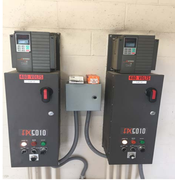
Image 3: Grinder Pump & Variable Frequency Drive Control
