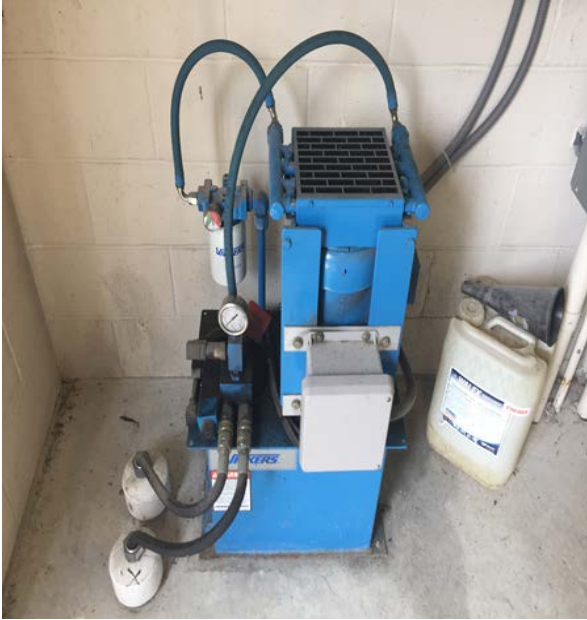
Image 3: Grinder Pump & Variable Frequency Drive Control
