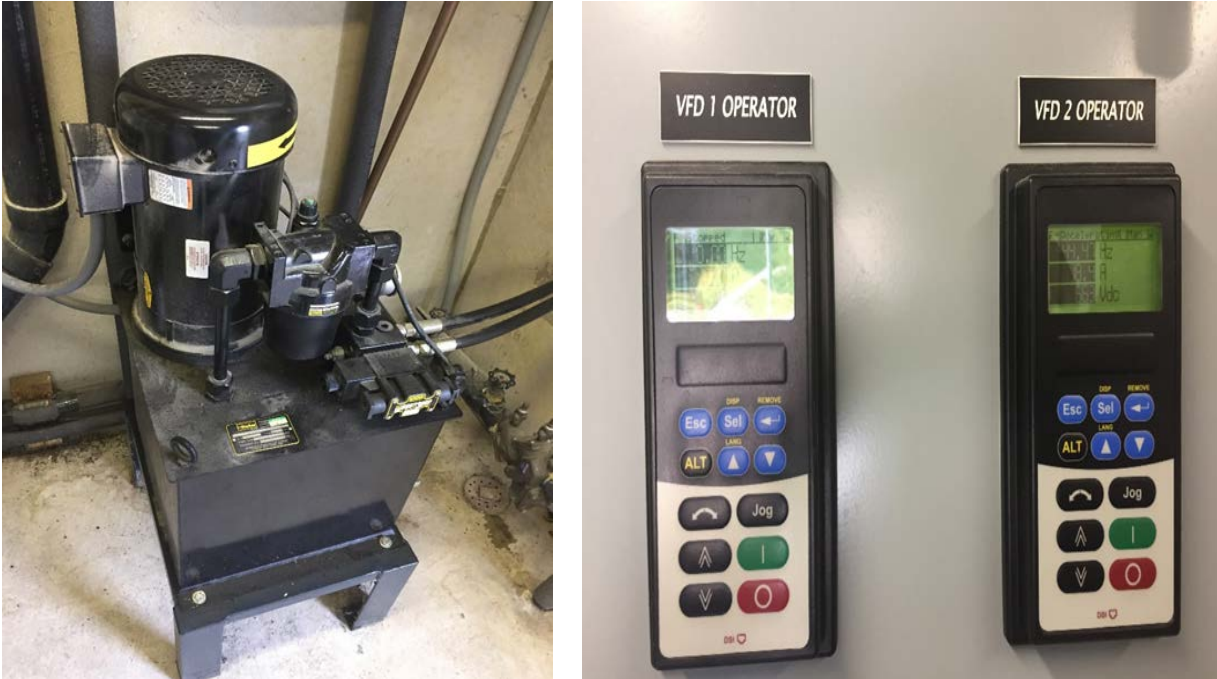
Image 5: Grinder Pump & Variable Frequency Drive Control System
