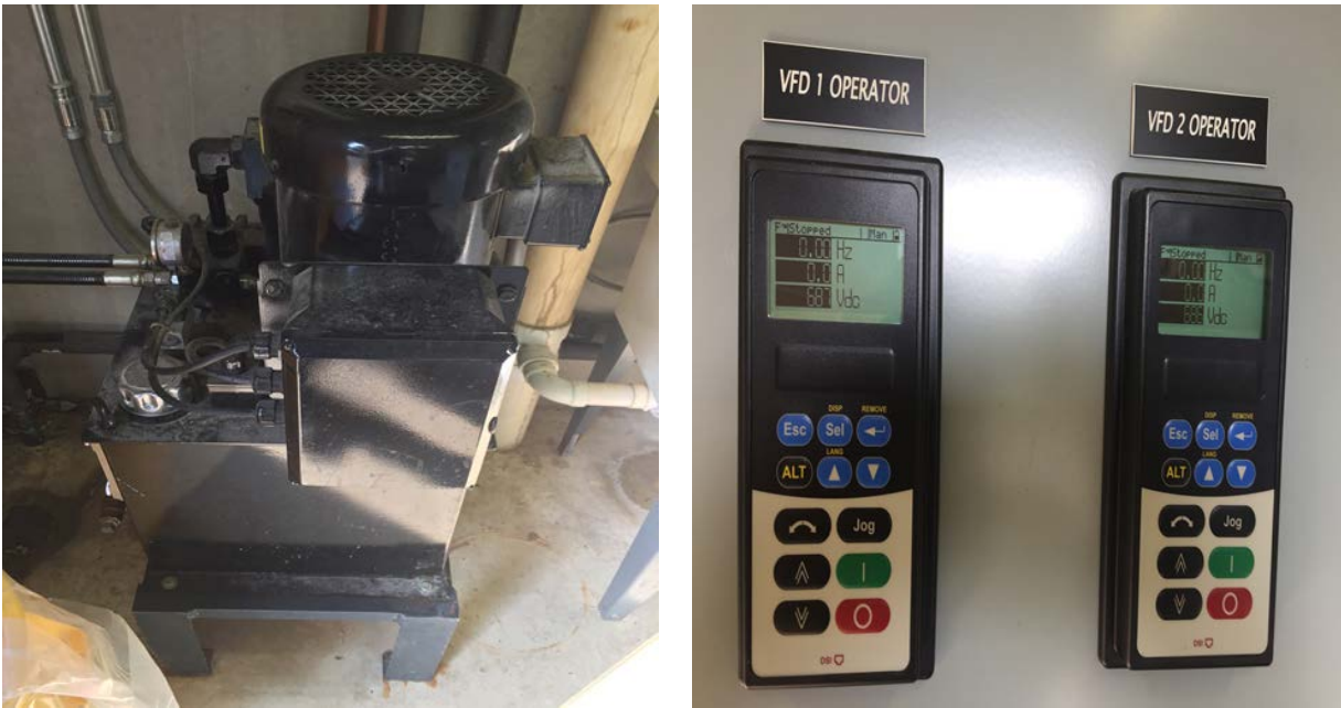
Image 5: Grinder Pump & Variable Frequency Drive Control System
