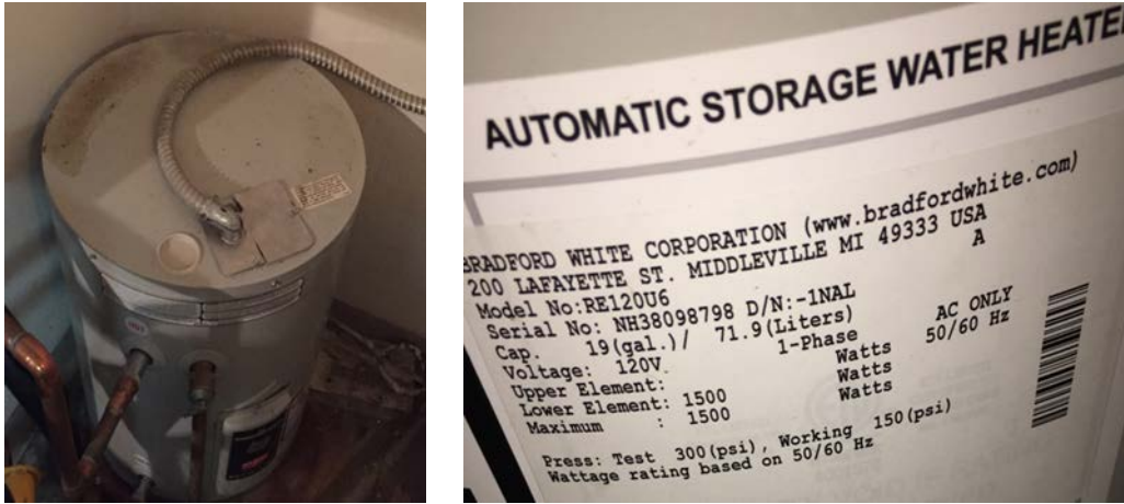
Image 6: Domestic Hot Water System
