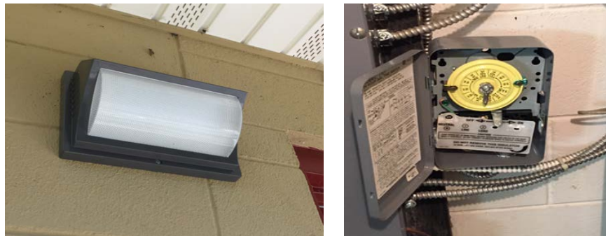
Image 3: Exterior Lighting & Timer
