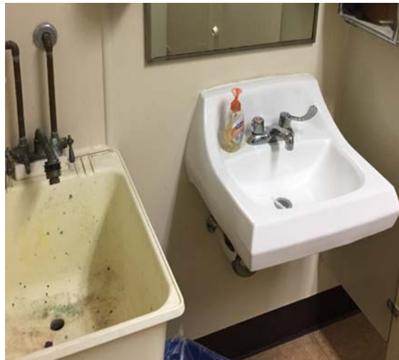
Image 7: Typical Restroom Faucets
