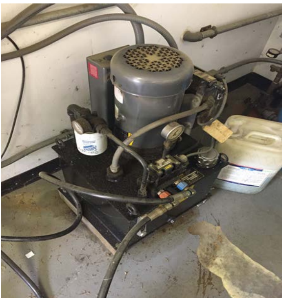
Image 4: Hydraulic Grinder Pump & Exhaust Fan
