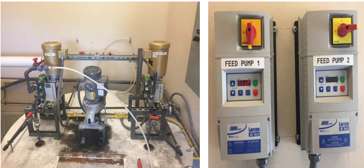
Image 5: Feed (Lime) & Mixing Pumps
