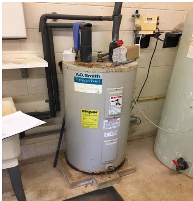
Image7: Domestic Water Heater
