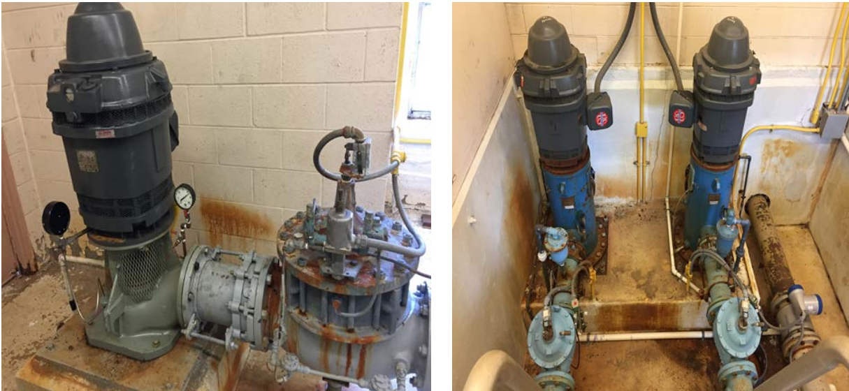
Image 4: Main & Booster Pumps
