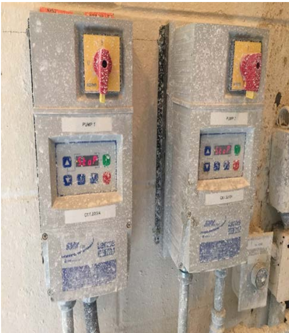
Image: VFDs and Water Treatment Tanks
