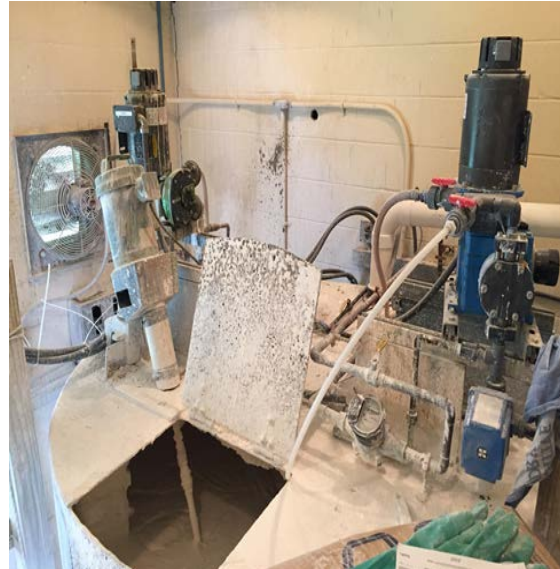
Image 1: Well Pump, and Lime and Mixing Pumps
