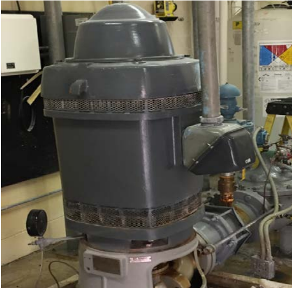
Image 1: Well Pump, and Lime and Mixing Pumps
