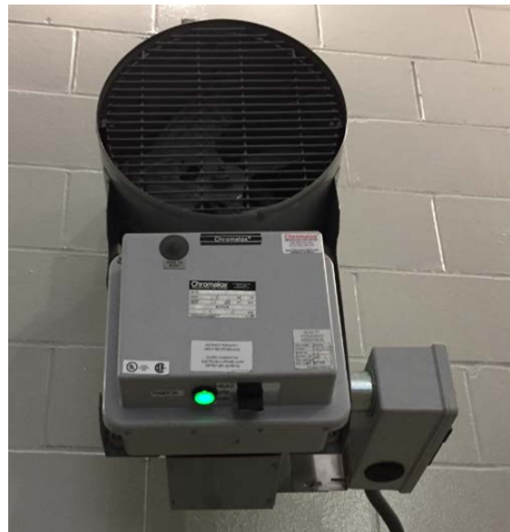
Image 5: Dehumidifier and Line Voltage Thermostat
