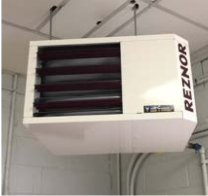
Image 3: Gas Fired Unit Heater and Thermostat
