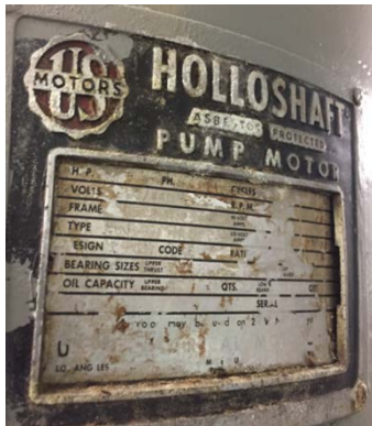
Image 5: Well Pump Name Plate & Chlorine Pump
