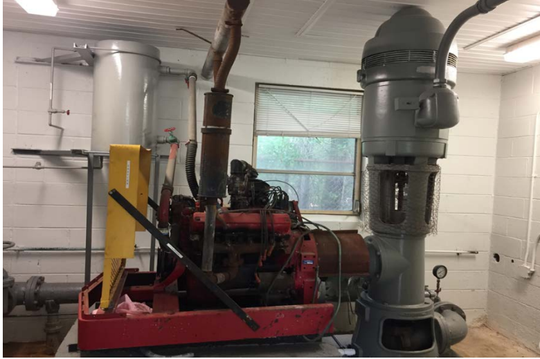
Image 4: 75 hp Well Pump, with natural Gas Fueled Engine
