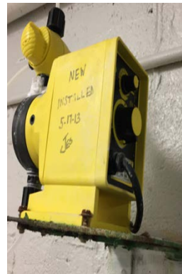
Image 5: Well Pump Name Plate & Chlorine Pump
