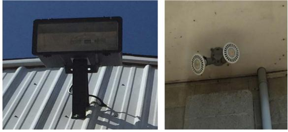
Image 3: Exterior Metal Halide (left) and LED (right) Fixtures
