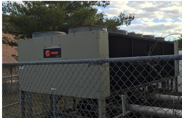
Image 5: Trane Chilled Water System and Related Equipment
