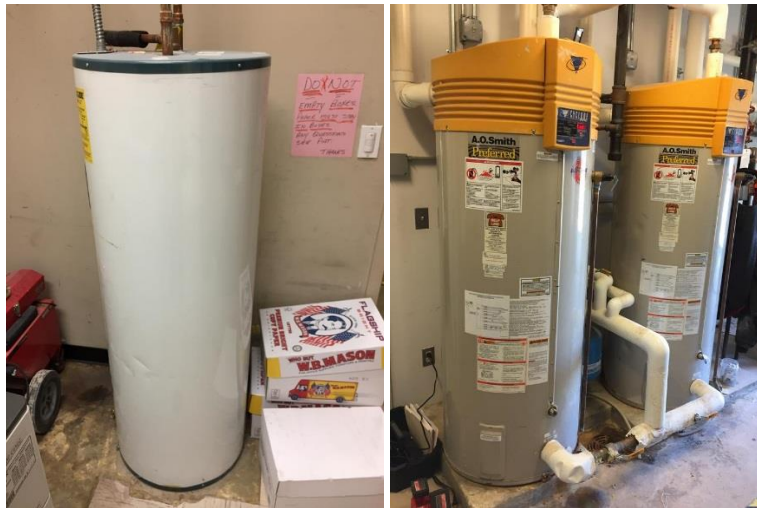
Image 6: One Electric DHW Heater and Two Gas-Fired DHW Heaters
