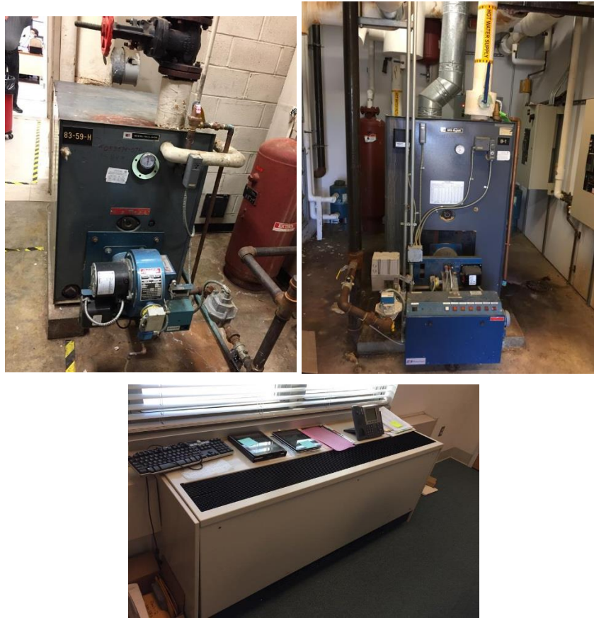
Image 3: Hot water boilers and unit ventilators
