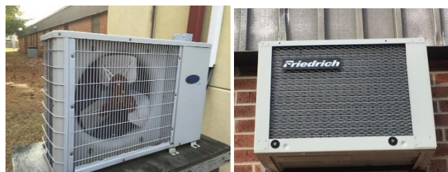
Image 4: Ductless Mini-Split and Through-the-wall AC units
