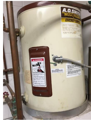
Image 4: Domestic Hot Water Heating
