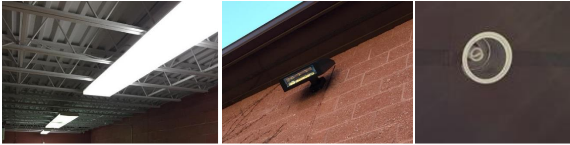
Image 2: Interior and Exterior Lighting Fixtures
