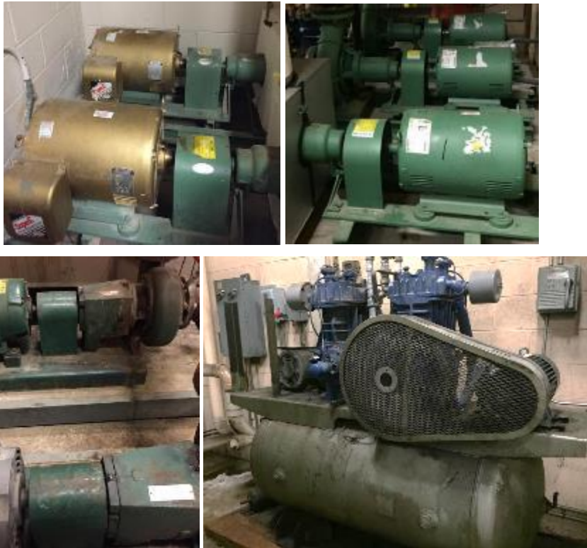
Image 5: Newer chilled water pumps and older hot water pumps and compressors
