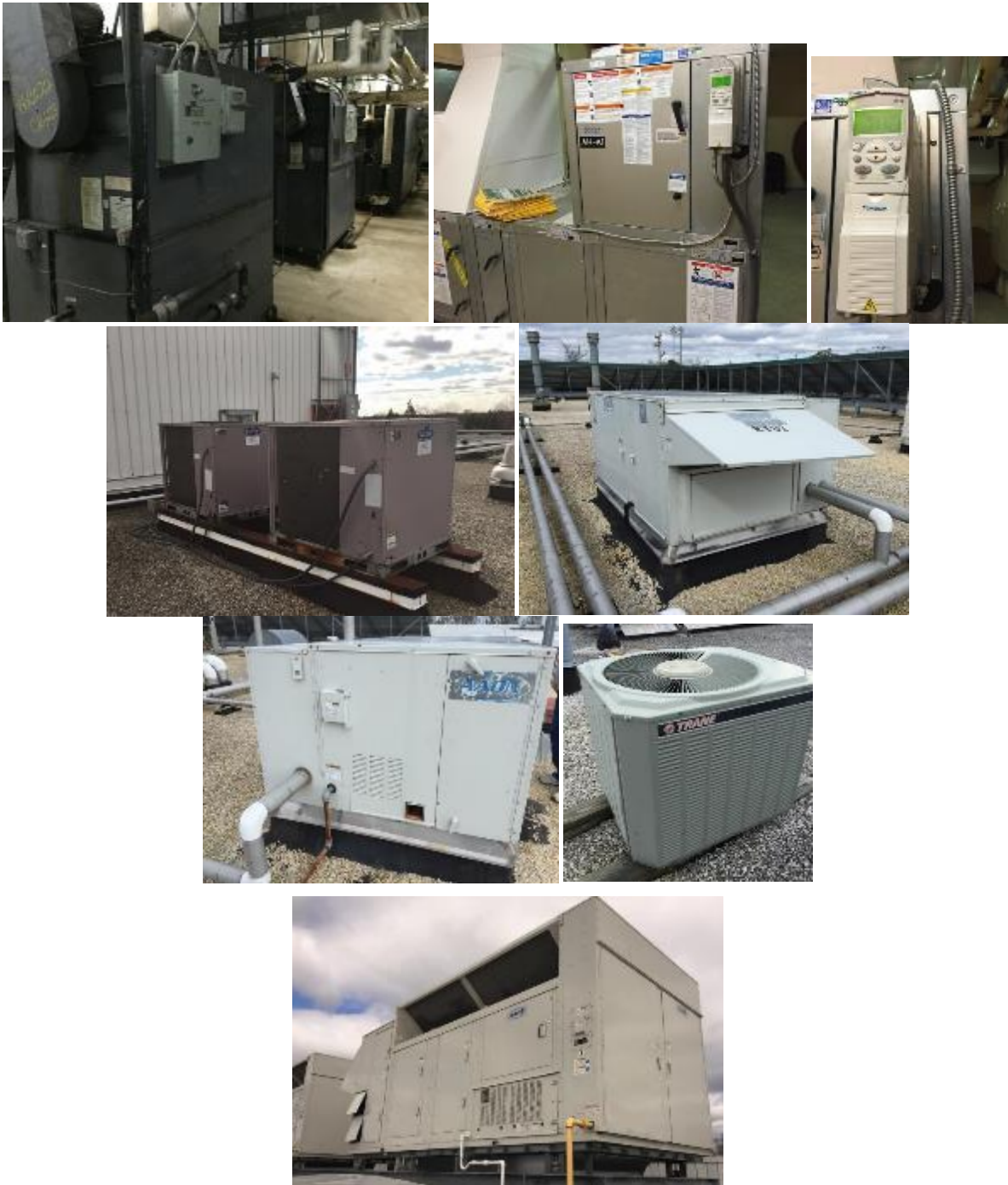
Image 6: Air handling units, packaged RTUs, and split systems
