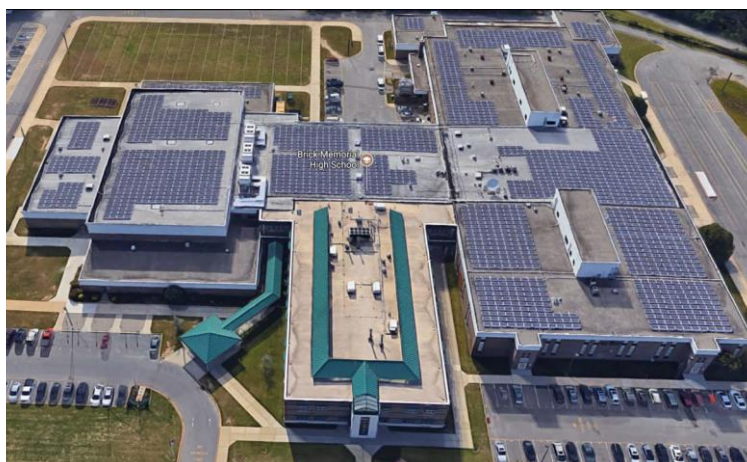
Image 11: Aerial view of BMHS showing solar array
