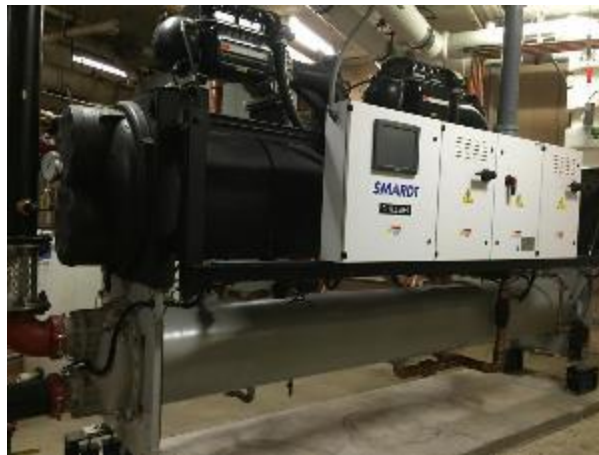
Image 3: Chillers and Cooling Towers
