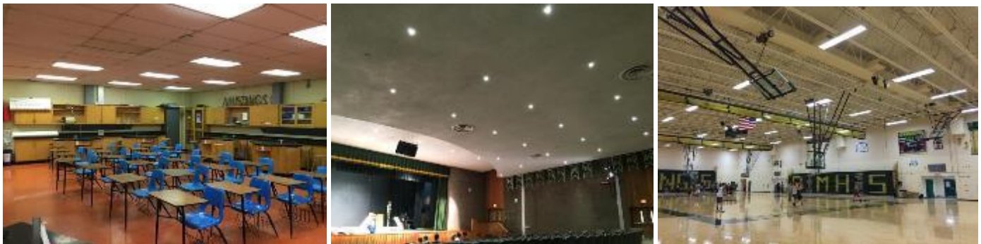
Image 2: Building Interior and Exterior Lighting
