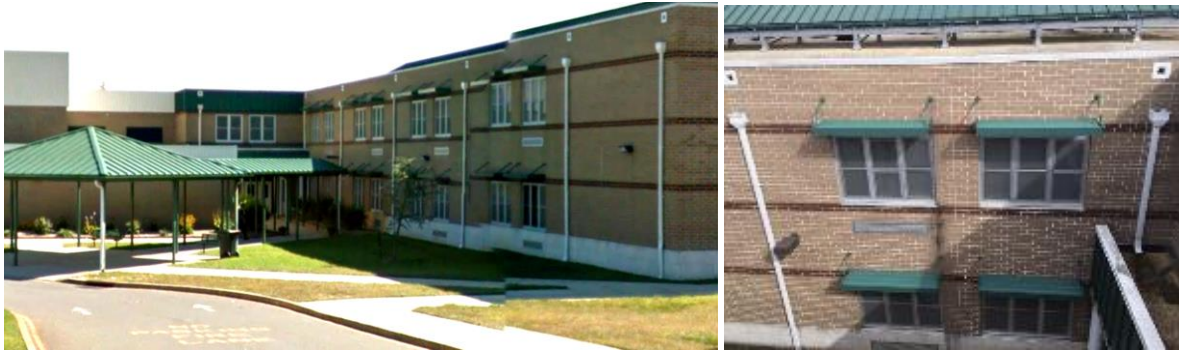
Image 1: BMHS front exterior walls and windows
