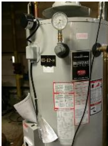
Image 8: Domestic hot water heater
