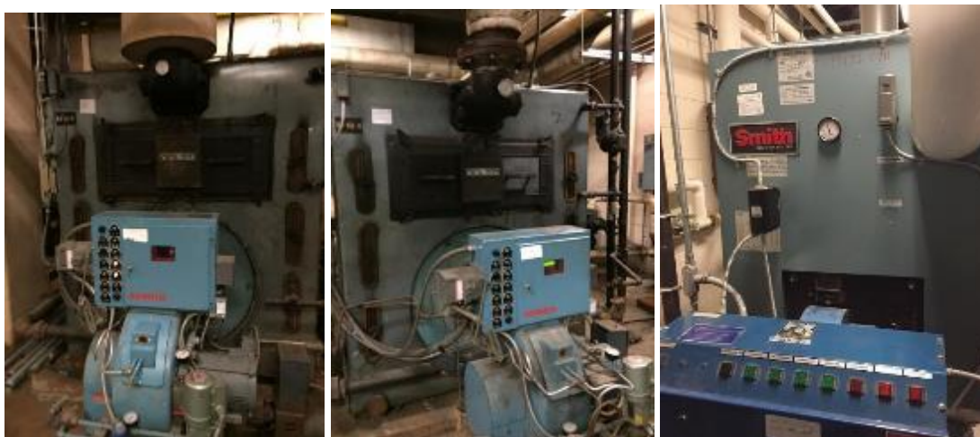
Image 4: Hot Water Boilers 1, 2 and 3
