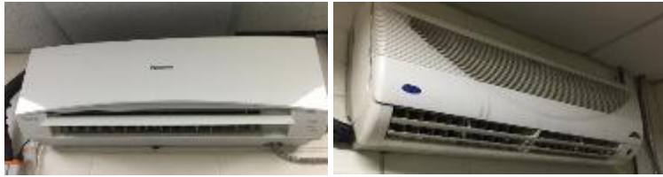
Image 7: Ductless mini-split systems
