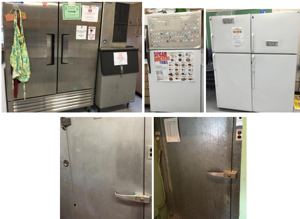
Image 6: Building Refrigeration Units
