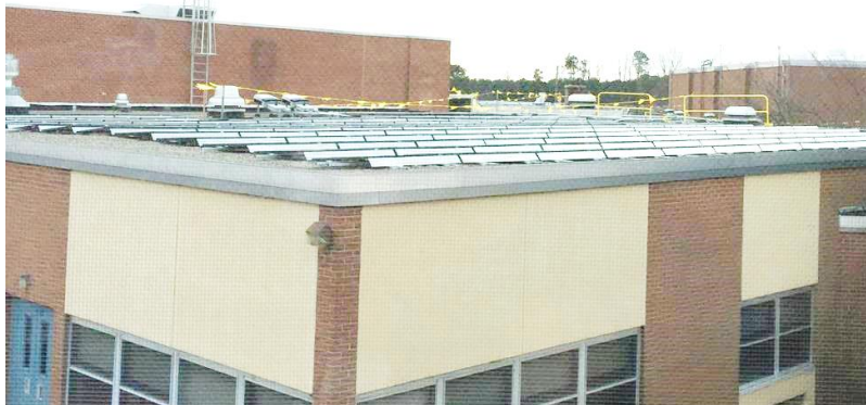
Image 1: Rooftop Solar PV Array Under Construction at LRMS
