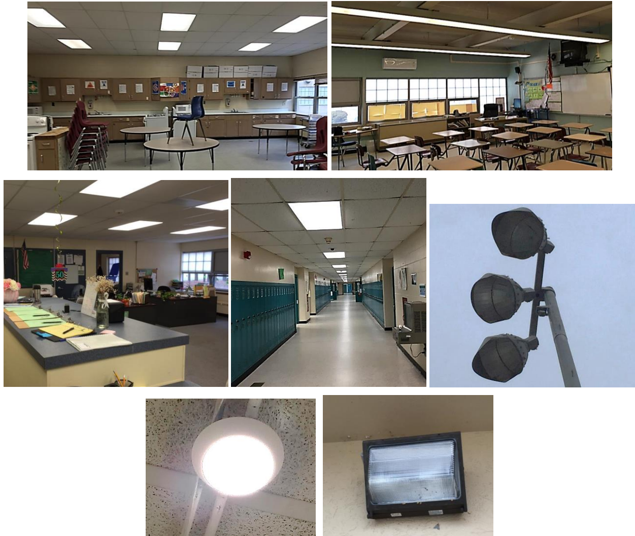
Image 2: Interior & Exterior Light Fixtures
