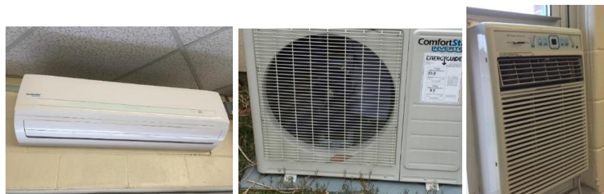
Image 5: Ductless Mini-Splits & Window AC Units provide most of the cooling to the building
