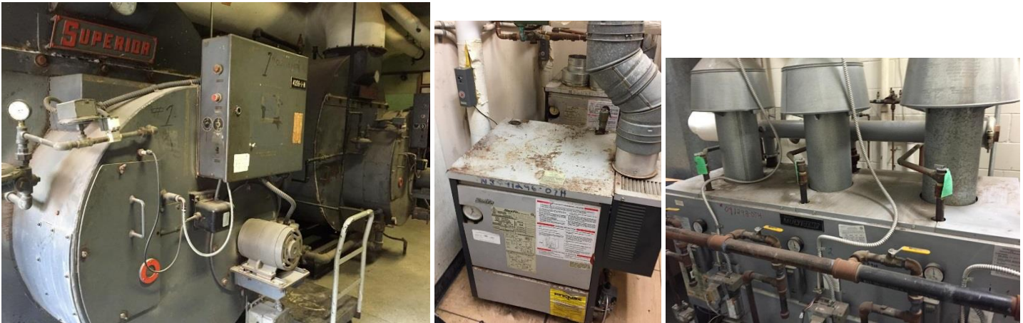
Image 3: Building Boiler Systems
