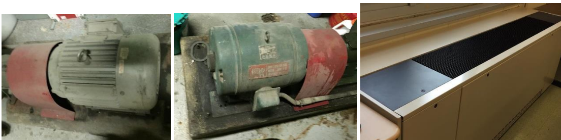
Image 4: Heating hot water pumps distribute hot water to unit ventilators
