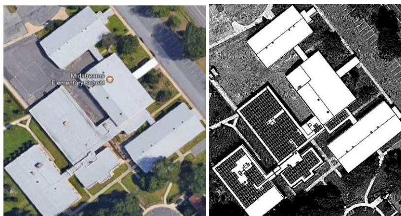
Image 10: School’s rooftop before and after solar PV installation
