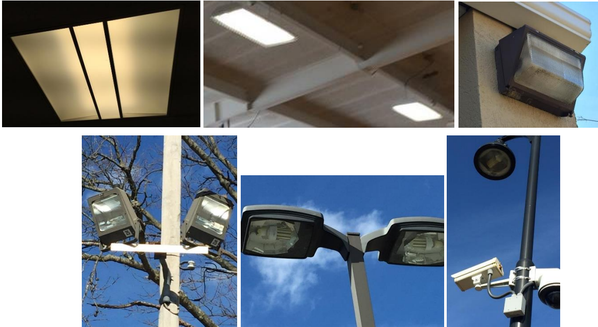
Image 2: Building Interior & Exterior Lighting
