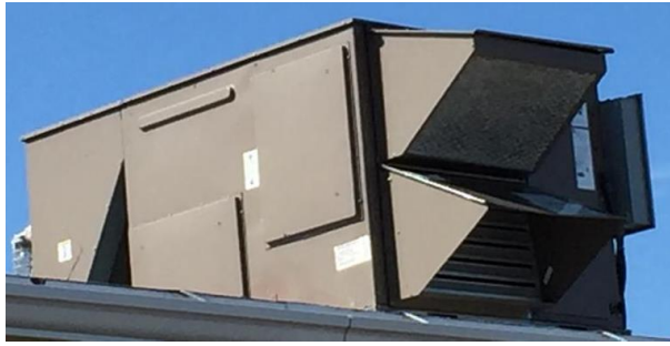
Image 5: York RTU on roof above the Library
