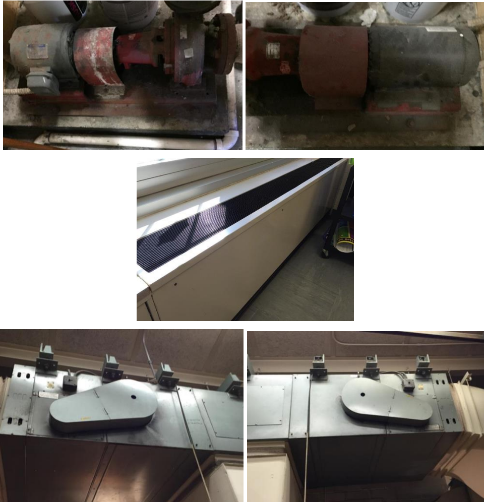
Image 4: Heating Hot Water Pumps, Classroom Unit Ventilators, AHUs in Multi-Purpose Room
