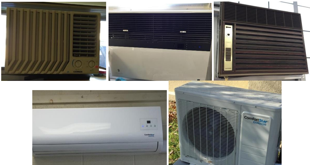
Image 6: A mix of old window AC units & some newer, high efficiency ductless mini-split AC units supply building cooling
