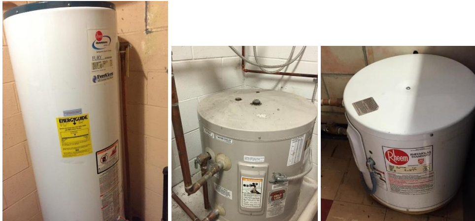
Image 7: Domestic Hot Water Heaters
