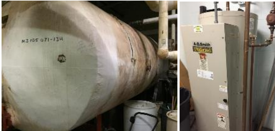
Image 6: Domestic hot water heater and large DHW storage tank.
