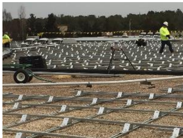
Image 2: Rooftop solar PV array under construction at VMMS (Feb 22, 2017)
