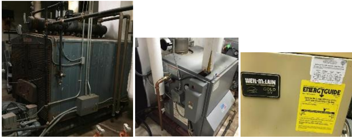
Image 4: Building heating is provided by 2 large main boilers, 5 smaller boilers in the newer additions
