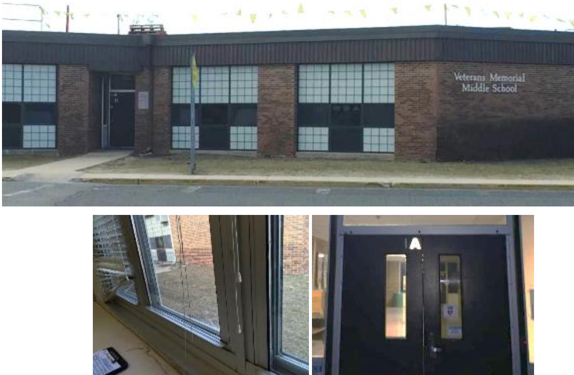
Image 1: Building front exterior, windows, and doors
