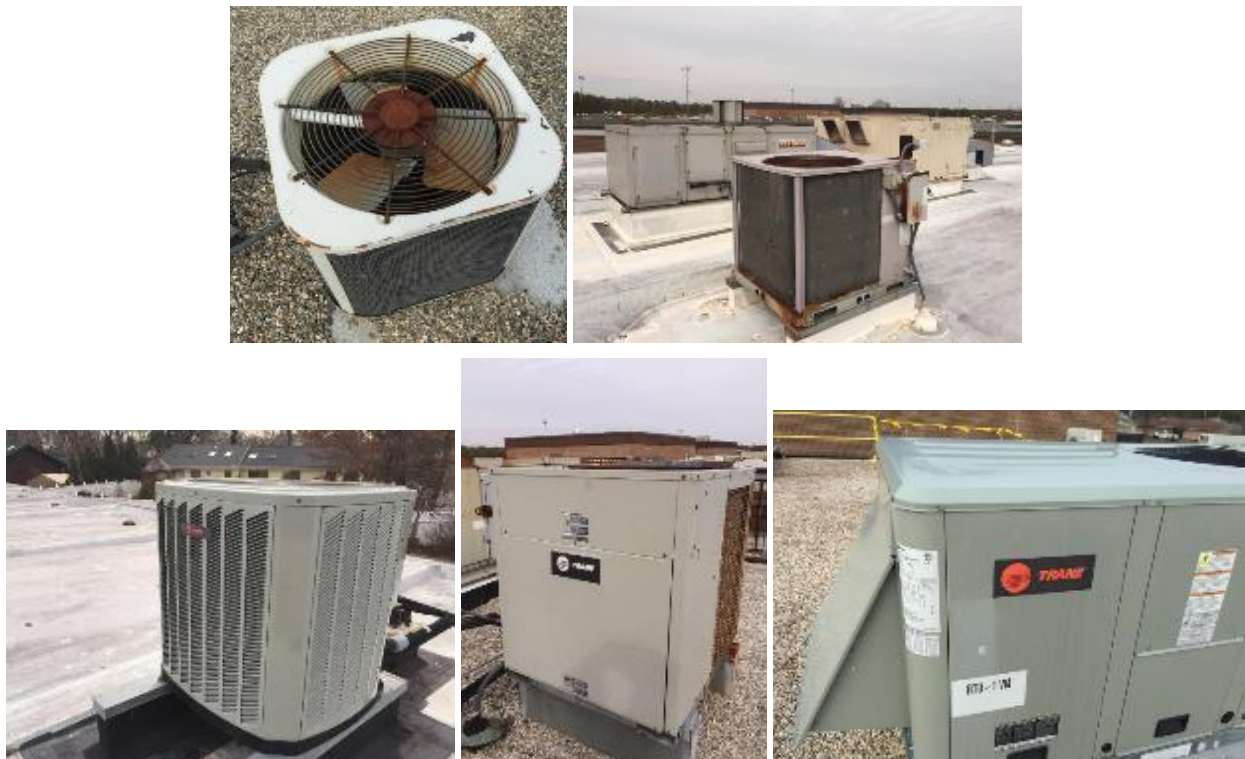
Image 5: Building cooling is provided by multiple RTUs, mini-split, and window AC units
