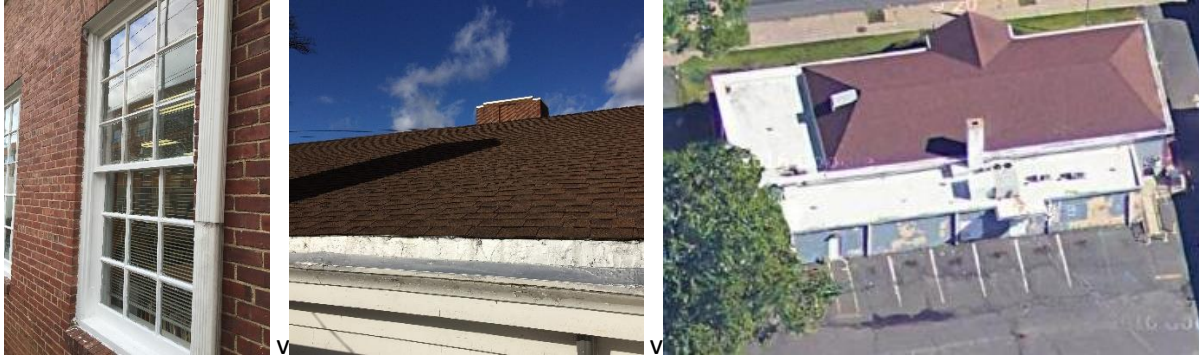
Image 1 Building envelope images
