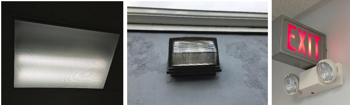
Image 2 Typical lighting fixtures
