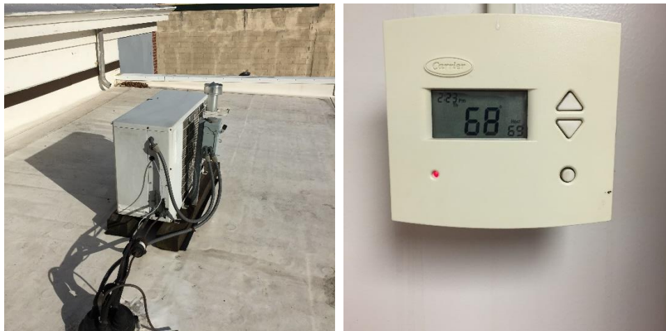
Image 4 Space cooling equipment with a sample thermostat
