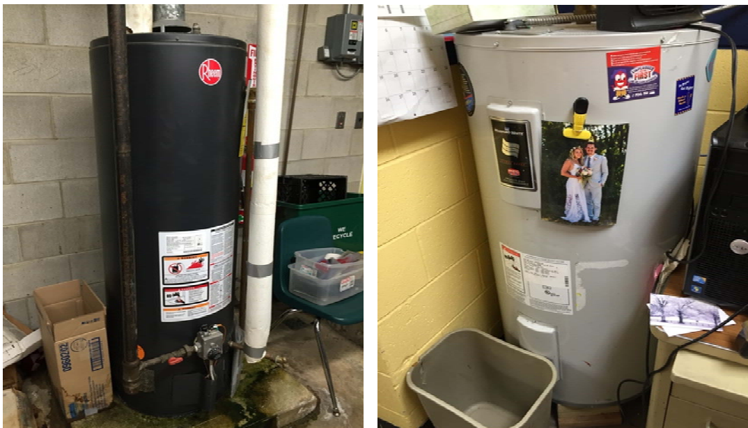
Image 6 Domestic hot water heaters serving the kitchen and the restrooms
