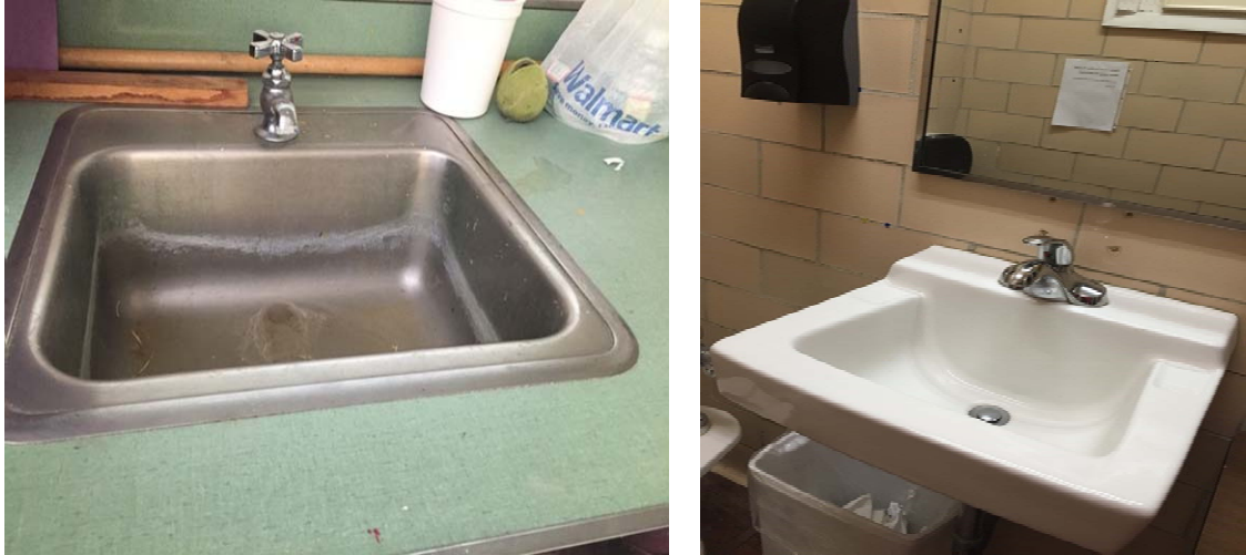
Image 9 Sample of sinks in the classrooms and restrooms
