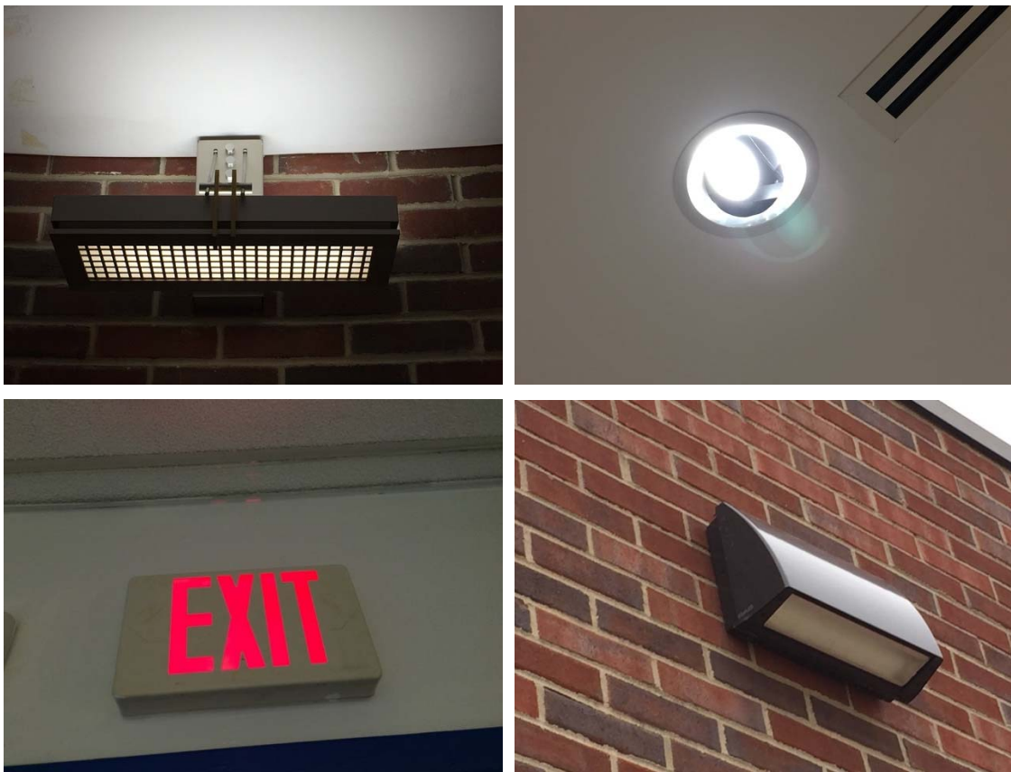
Image 2 Typical lighting fixtures
