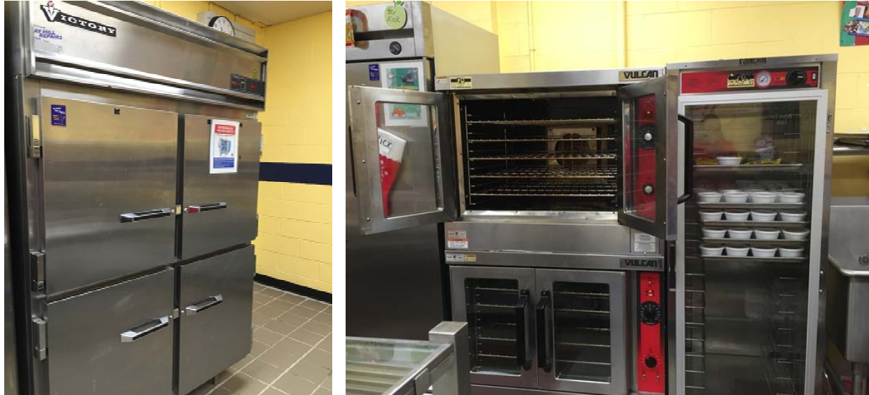
Image 7 Refrigeration and cooking equipment sample
