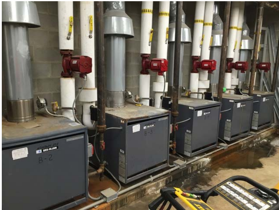
Image 3 Hot water boilers
