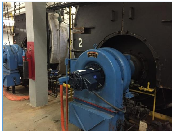
Image 3 Hot water boiler
