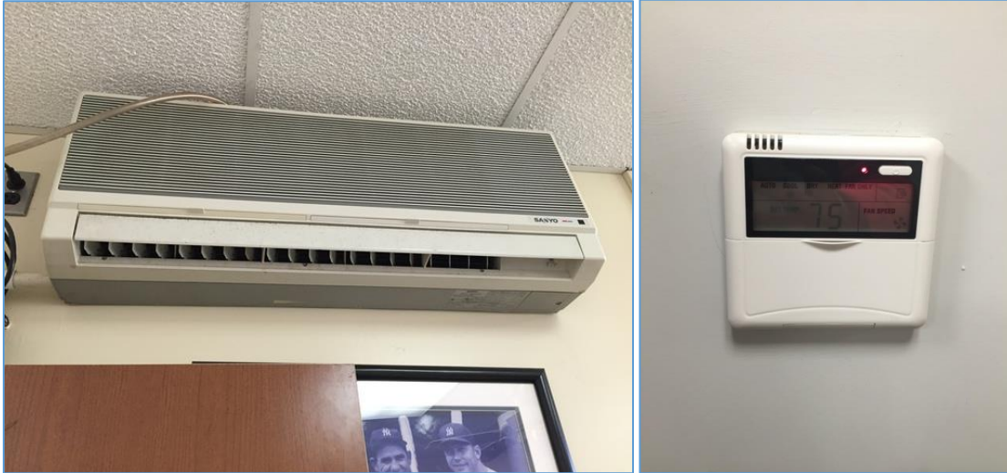
Image 4 Split AC system; Programmable thermostat
