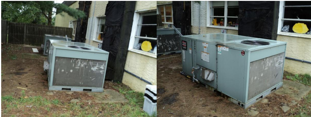
RTU's # 9 and 10 (L.) and RTU # 9
