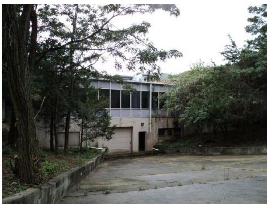
Partial North Façade
