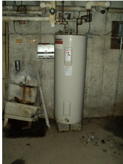
Electric DHW heater
