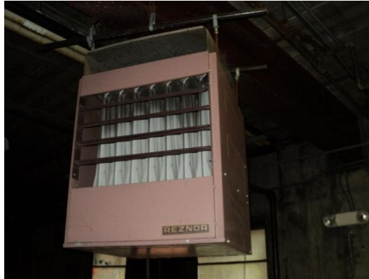
Basement Unit Heater
