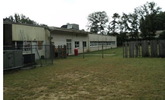
Partial West Façade
