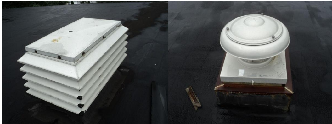
Typical roof mounted exhaust fans
