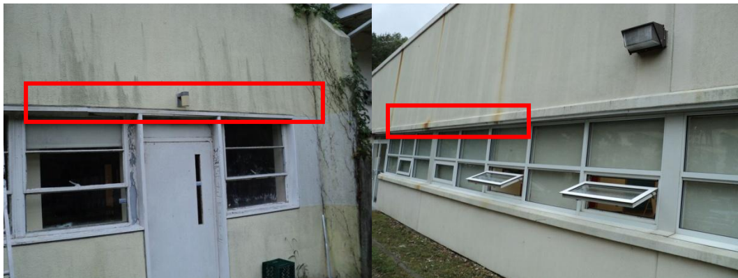
Damaged window frames, missing window sill and drip-edge details, signs of both exterior and interior mold and water damage around windows
