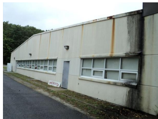
Partial South Façade
