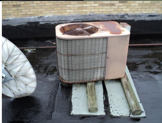
Comfort Star DX split system serving the library (above) and Zone # 1 condenser
