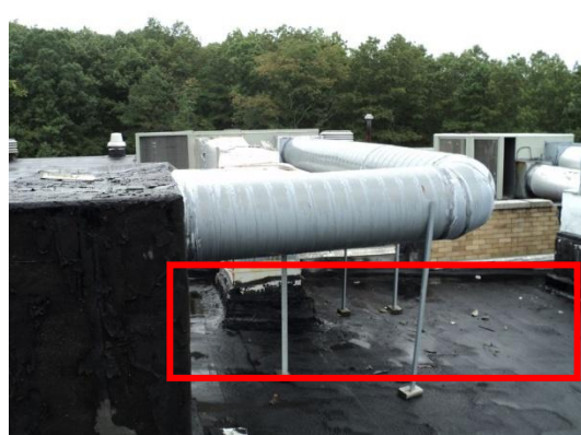
Signs of standing water and pooling, uncontrolled roof water run-off due to defective/clogged gutters and downspouts, cracking and bubbling of the membrane surface and the presence of loose sharp objects on the roof surface.
