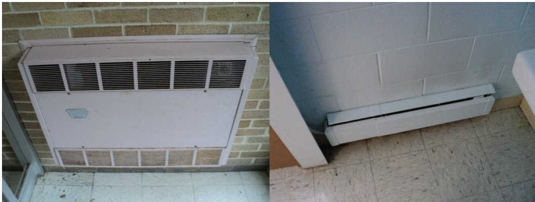
Electric heating equipment
