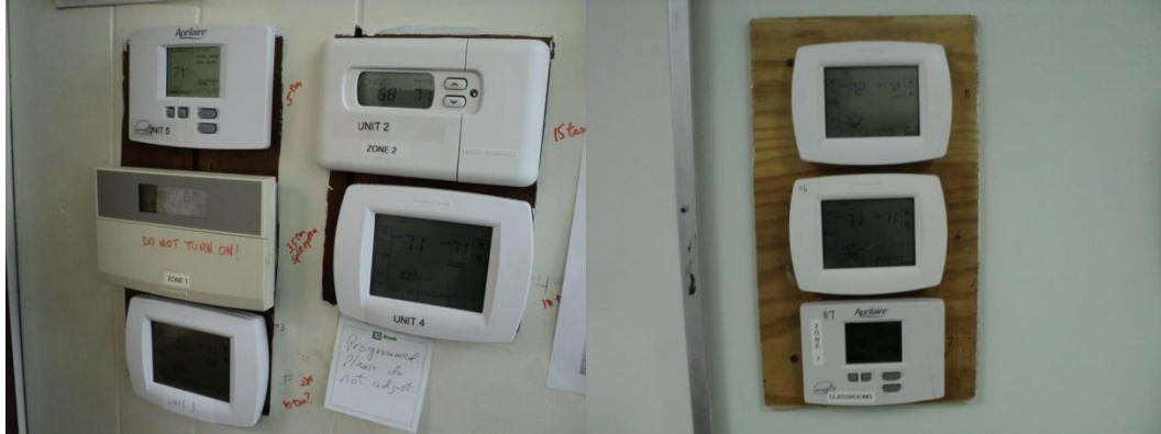
Typical digital programmable thermostats
