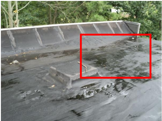
Signs of standing water and pooling, uncontrolled roof water run-off due to defective/clogged gutters and downspouts, cracking and bubbling of the membrane surface and the presence of loose sharp objects on the roof surface.
