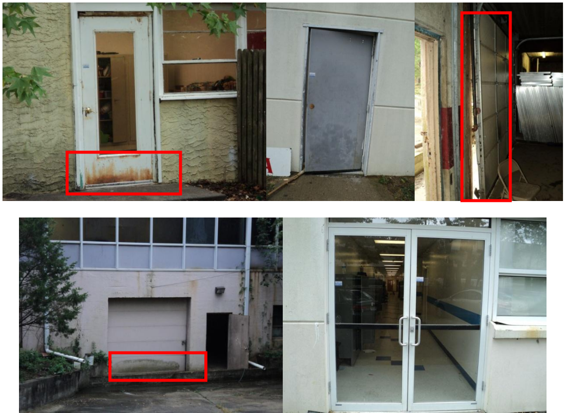
Signs of a damaged solid metal with glass panel door and a damaged and warped overhead door frame. SWA also observed that un-insulated doors were installed between different conditioned spaces and missing and worn weather-stripping
