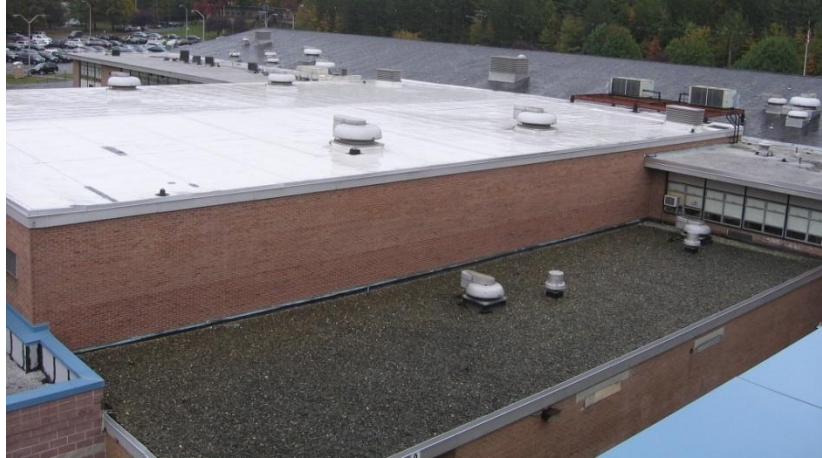
Image shows 4 different roofing materials
