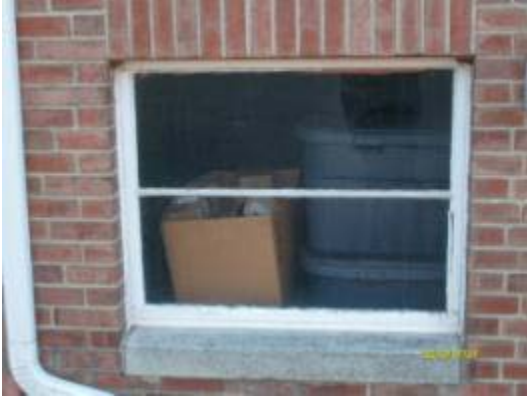
Exposed and damaged frames that are major sources of thermal bridging
