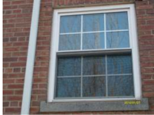
Exposed and damaged frames that are major sources of thermal bridging
