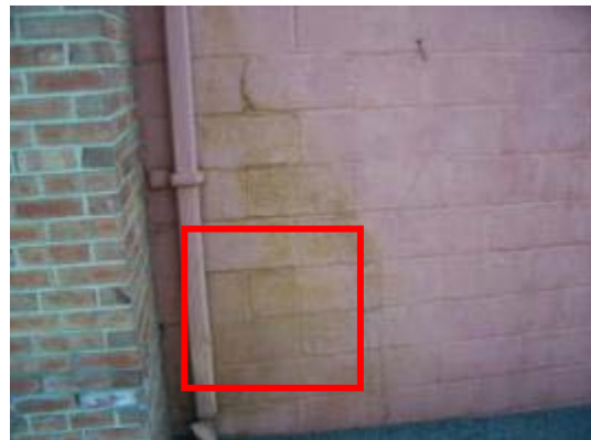
Examples of cracked and missing caulk and signs of water damage
