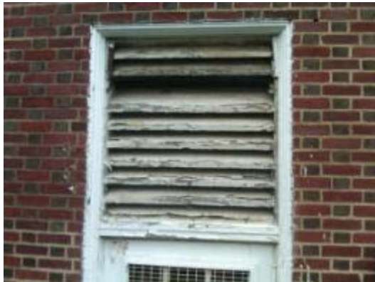
Signs of water damage at perimeter walls due to / ineffective site drainage and un-caulked/un-sealed exterior wall penetrations
