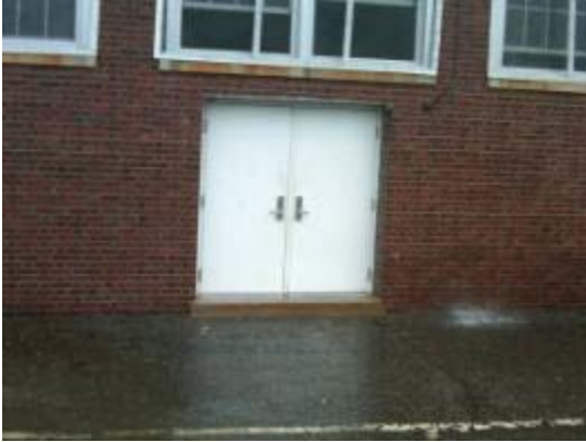
Damaged and aged door frames, missing/worn weather stripping
