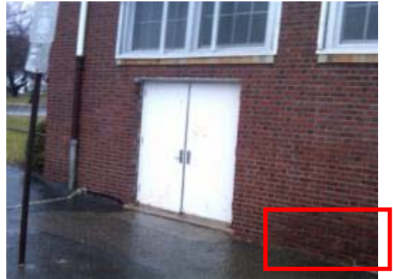
Signs of water damage at perimeter walls due to / ineffective site drainage and un-caulked/un-sealed exterior wall penetrations
