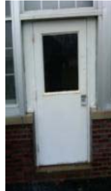
Damaged and aged door frames, missing/worn weather stripping
