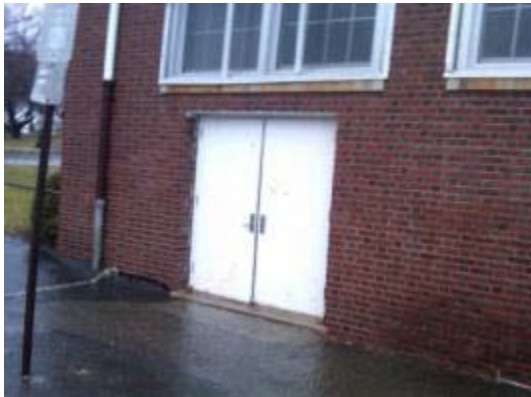
Partial South Façade
