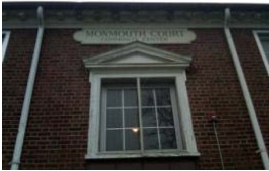
Partial West Façade
