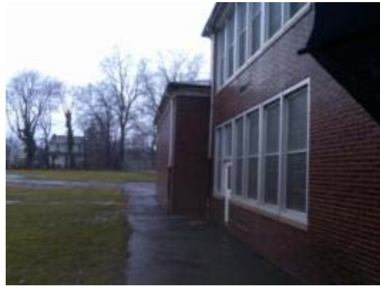
Partial East Façade
