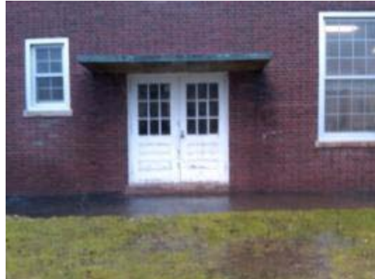
Partial North Façade
