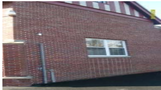
Partial West Façade
