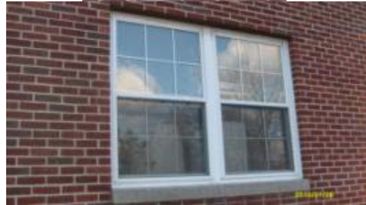
Exposed and damaged frames that are major sources of thermal bridging
