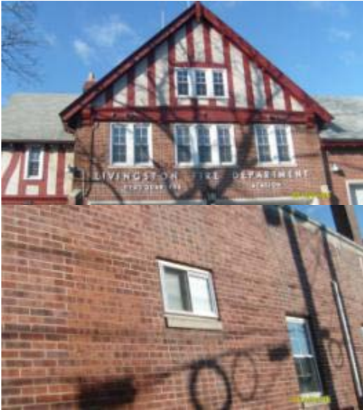
Exposed and damaged frames that are major sources of thermal bridging
