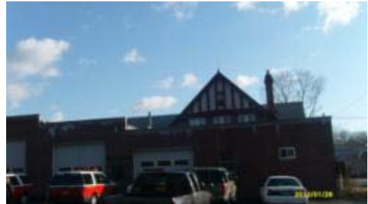
Partial West Façade
