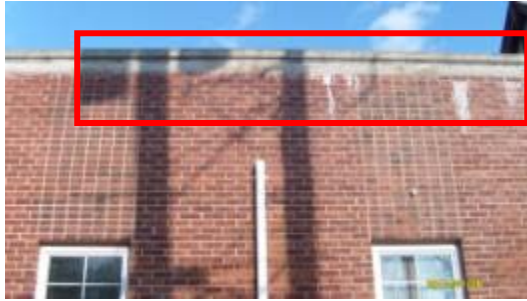
Examples of cracked and missing caulk and un-sealed exterior wall penetrations
