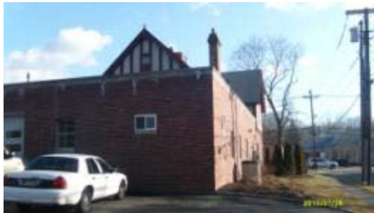
Partial South Façade
