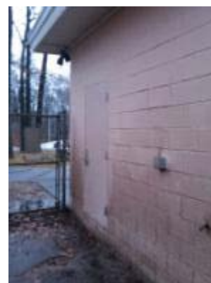
Partial West Façade
