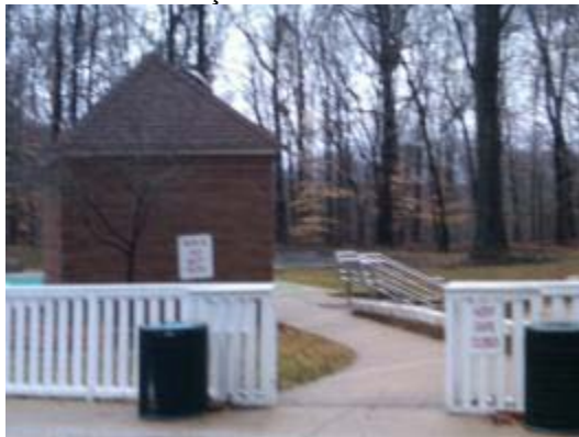
Children's Pool Pump House
