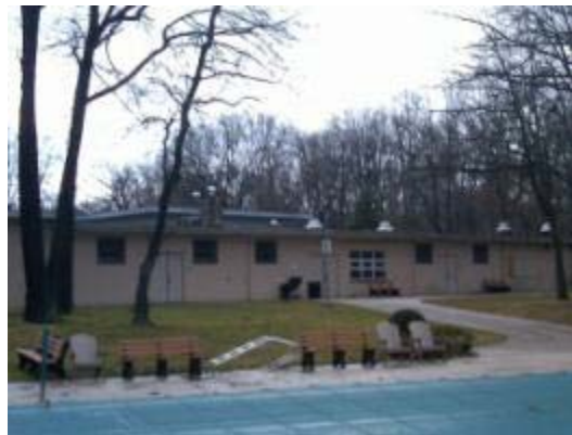
Partial North Façade
