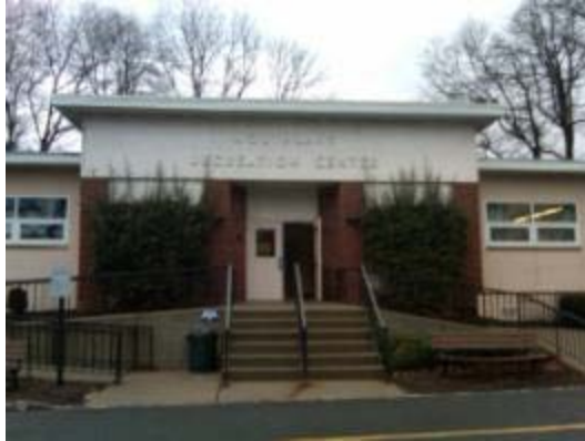
Partial South Façade
