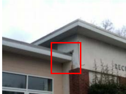
Missing/ ineffective flashing
