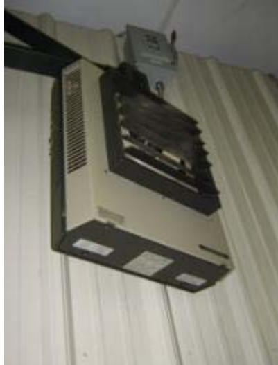
Electric unit heater
