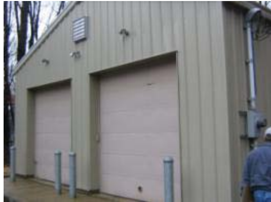
Overhead Doors on South Elevation
