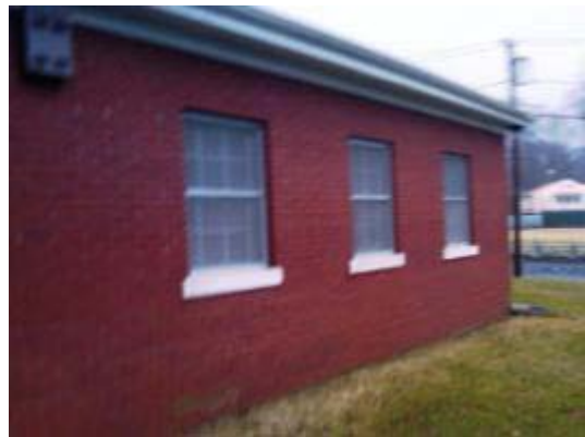
Partial East Façade
