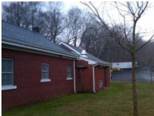
Partial North Façade
