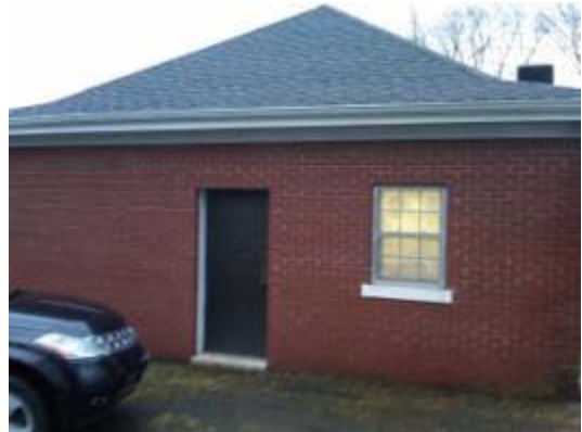
Partial West Façade
