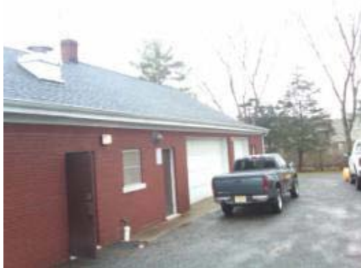
Partial South Façade
