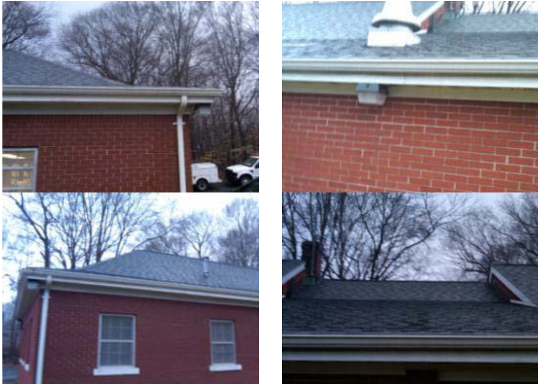
Typical roofing system throughout building
