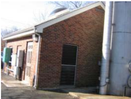
Building # 1 Front and Side Facade
