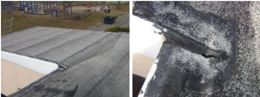
Roof of Deep Well; Roof Joint at Pool Building
